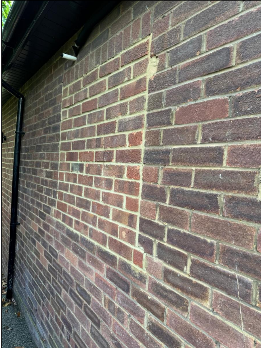
Figure 4: Photograph of the old bricks on the house.
