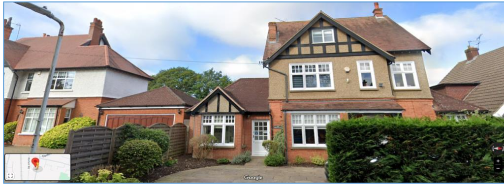
Figure 7: Image of varying roof treatments at numbers 23 & 25 Eastbury Road.
