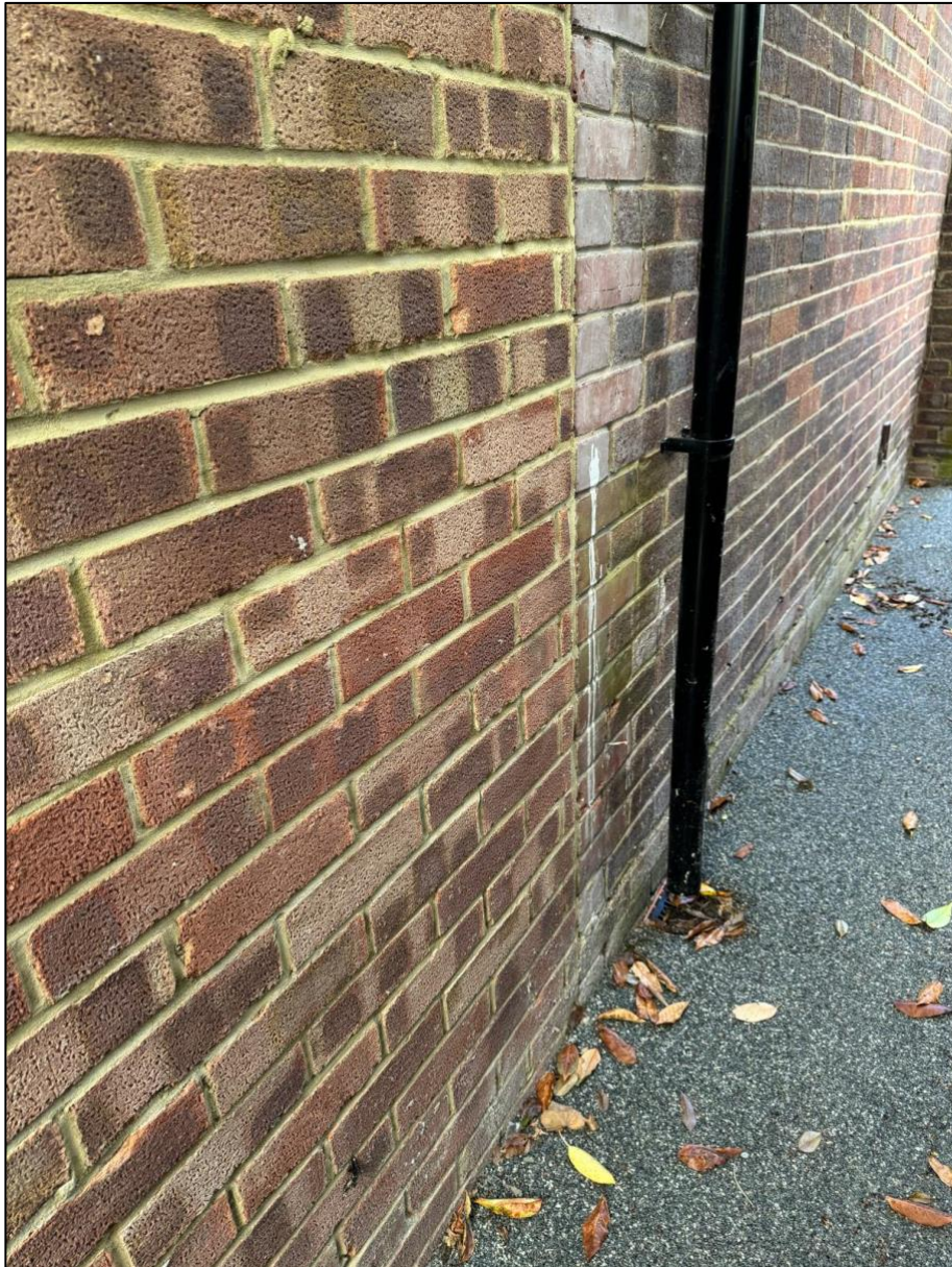
Figure 5: Photograph of the old bricks on the house.
