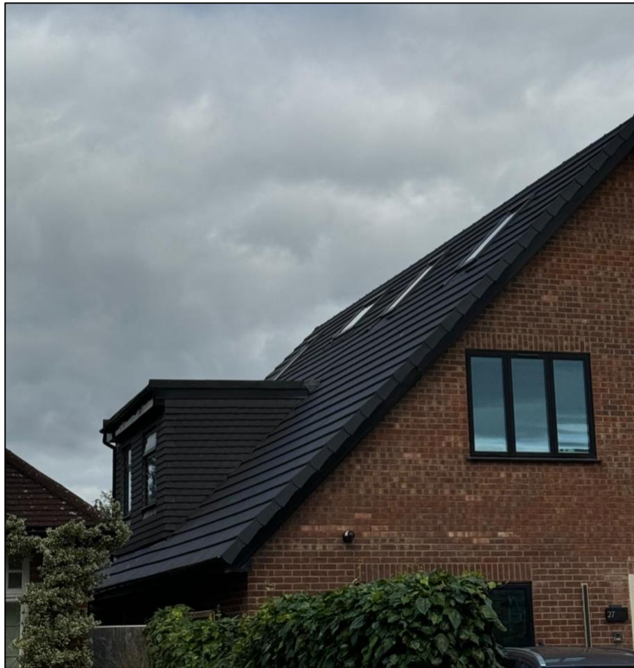
Figure 6: Photograph of the new rooftiles.
