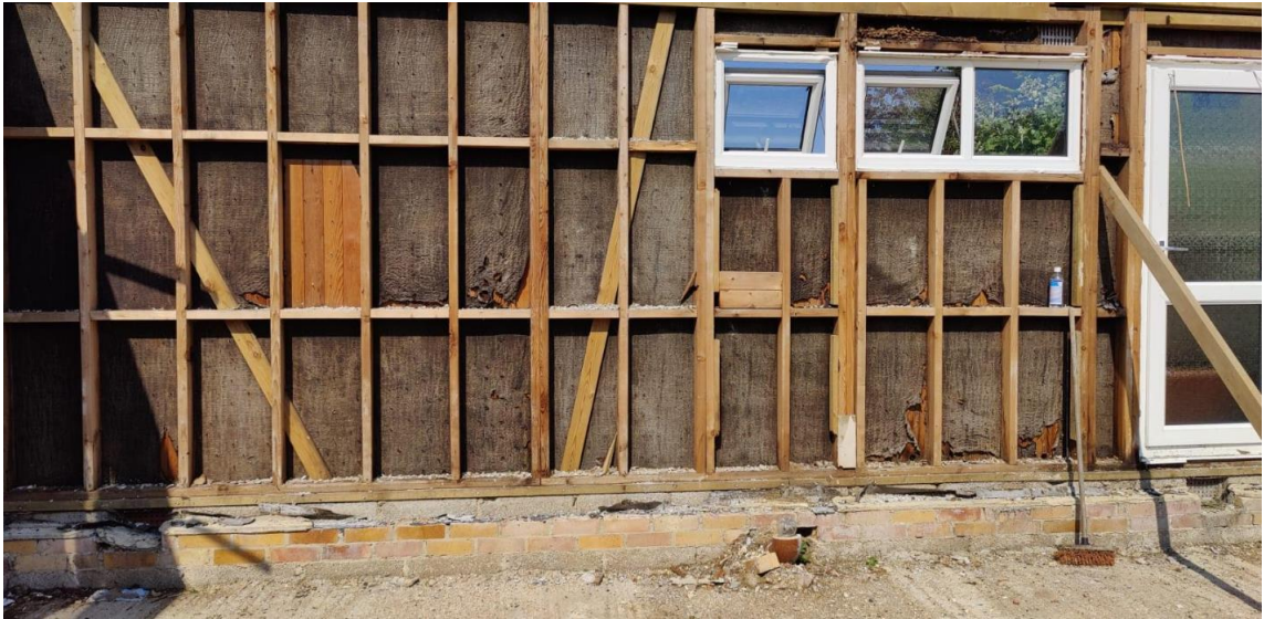
Existing stone clad timber building
