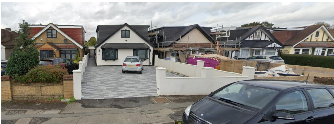
Flat roof dormers to properties on Pole Hill Road
