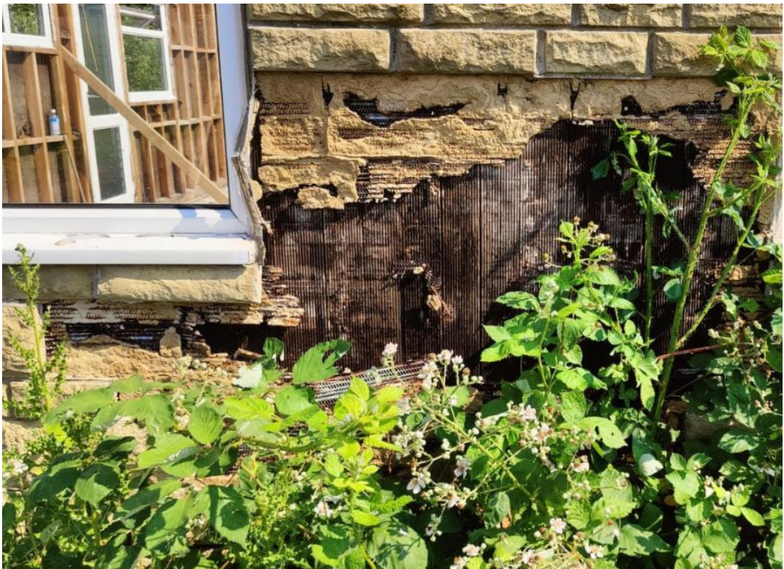
Existing stone clad timber construction
