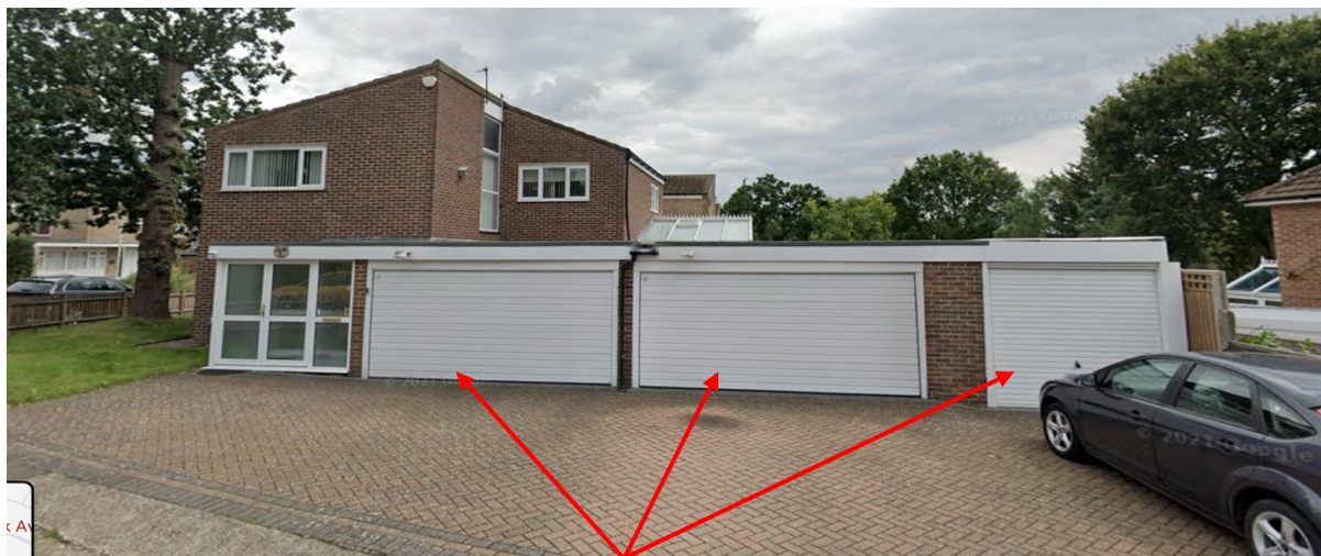
Figure 5 – 2 Roker Park Avenue 3 front garage doors
