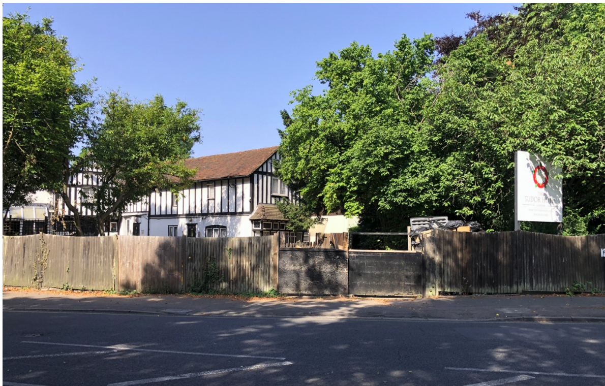
FIG. 2 – Existing boundary fencing at Field End Rd
