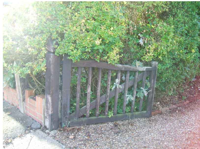
Original timber gate and post for chain link fence
