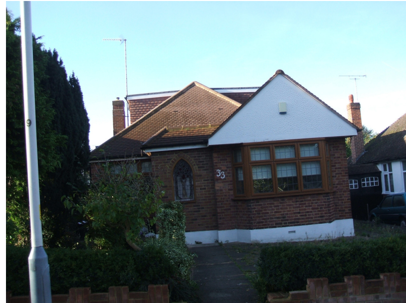
Altered property with roof additions
