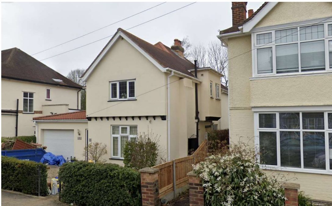
No 18 Myrtle Avenue – Detached two story houses with pitched roof. The roof height is lower than the adjoining houses.
