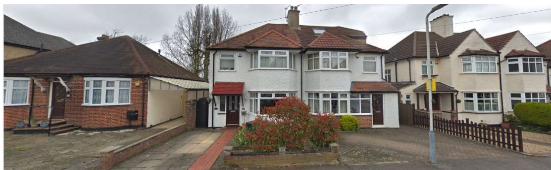
No 36 & 34 Myrtle Avenue – Pair of semi-detached houses with pitched roof.
