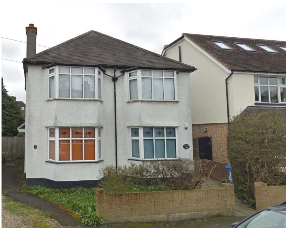
No 27 & 29 Myrtle Avenue – Pair of semi-detached houses with pitched roof.
