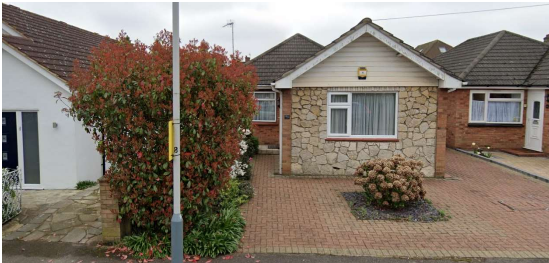
No 49 Myrtle Avenue – Detached bungalow with gable roof.
