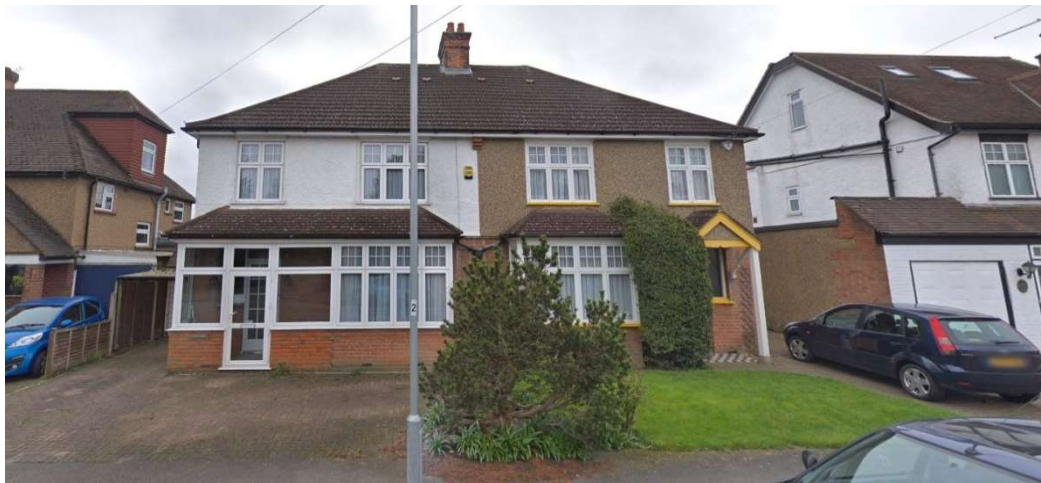
No 5 & 7 Myrtle Avenue – Pair of semi-detached houses with pitched roof.
