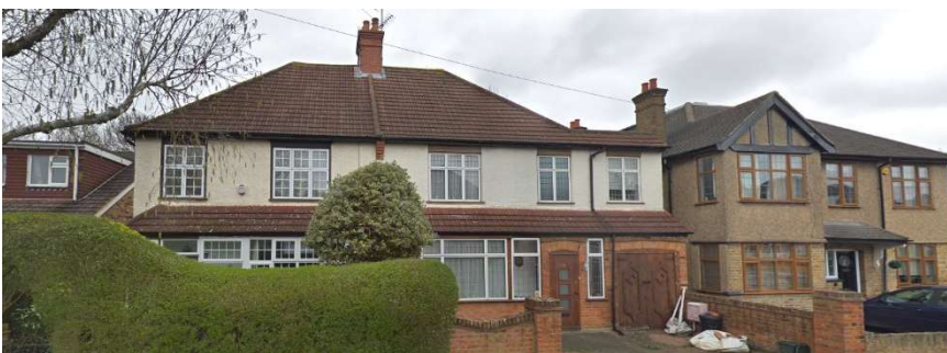
No 42 & 44 Myrtle Avenue – Pair of semi-detached houses with gable roof.
