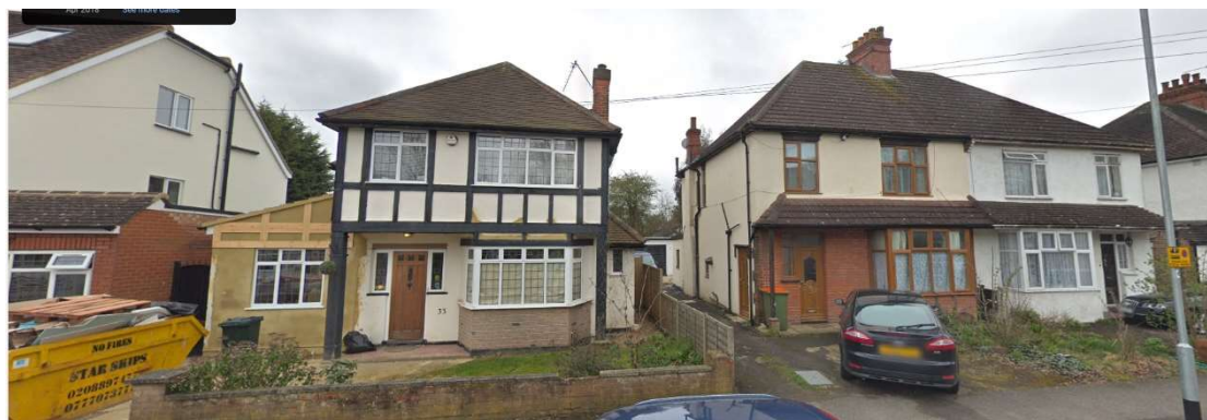
No 33 Myrtle Avenue – Detached two story houses with pitched roof.
