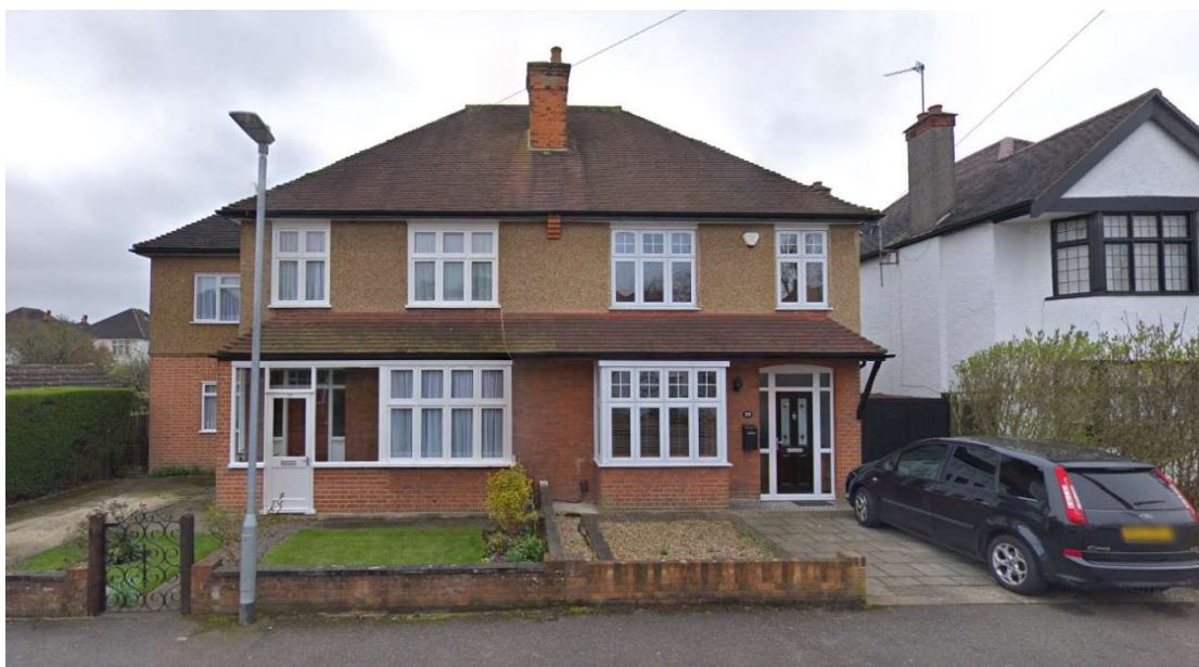
No 17 & 19 Myrtle Avenue – Pair of semi-detached houses with pitched roof.
