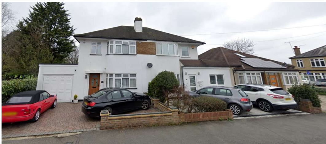
No 4 & 6 Myrtle Avenue – Pair of semi-detached houses with pitched roof.
