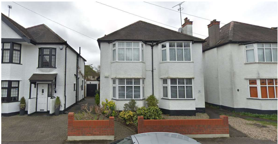
No 17 & 19 Myrtle Avenue – Pair of semi-detached houses with pitched roof.
