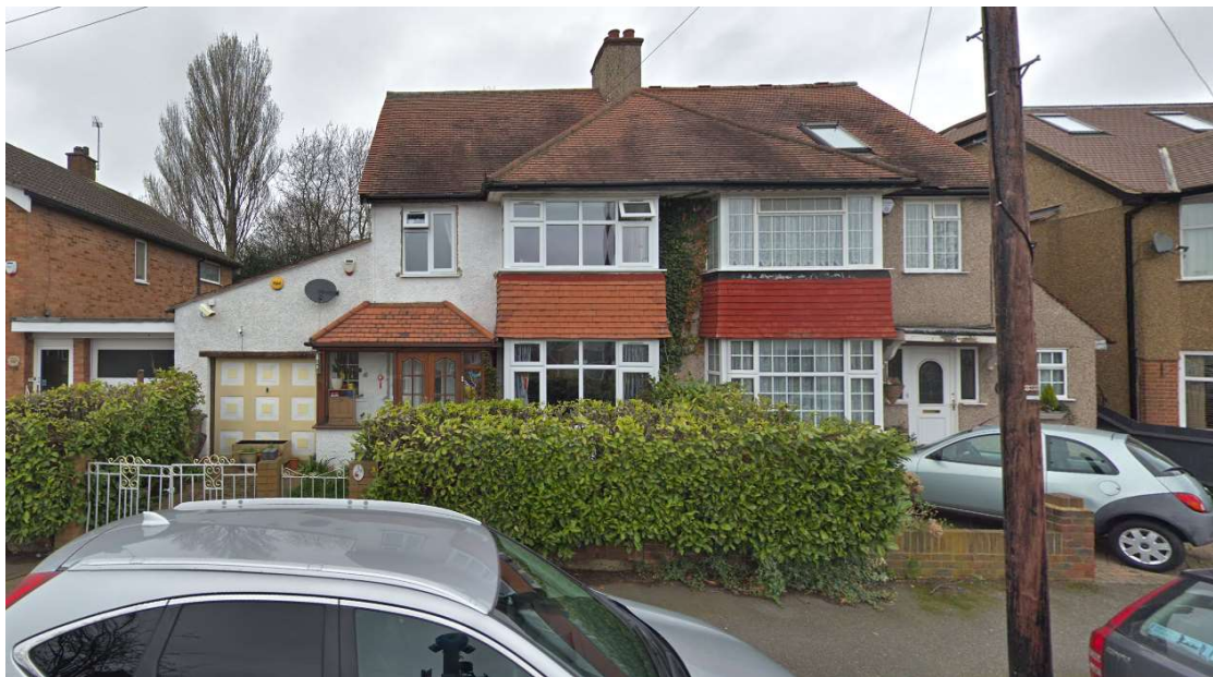
No 56 & 58 Myrtle Avenue – Pair of semi-detached houses with gable roof.
