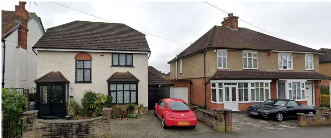
No 11 Myrtle Avenue – Detached two story houses with part gable and part pitched roof. The roof height is lower than the adjoining properties.
