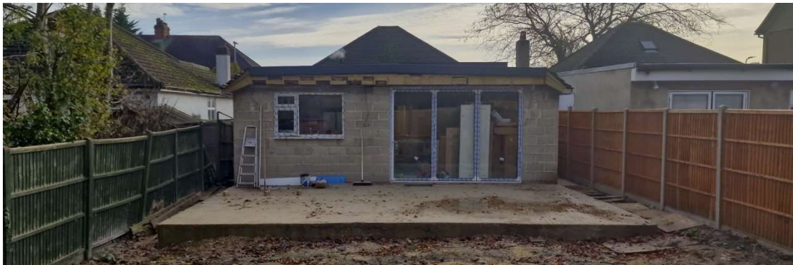
Existing Rear view of the property showing recently build 6M rear extension.
