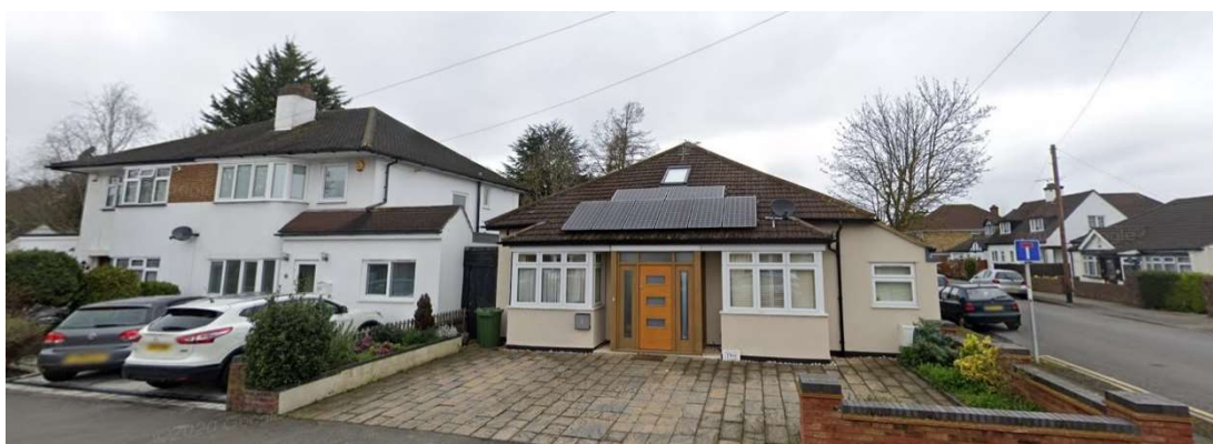
No 2 Myrtle Avenue – Detached bungalow with gable roof situated at the corner.
