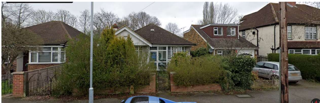
No 46 Myrtle Avenue – Detached bungalow with pitched roof.
