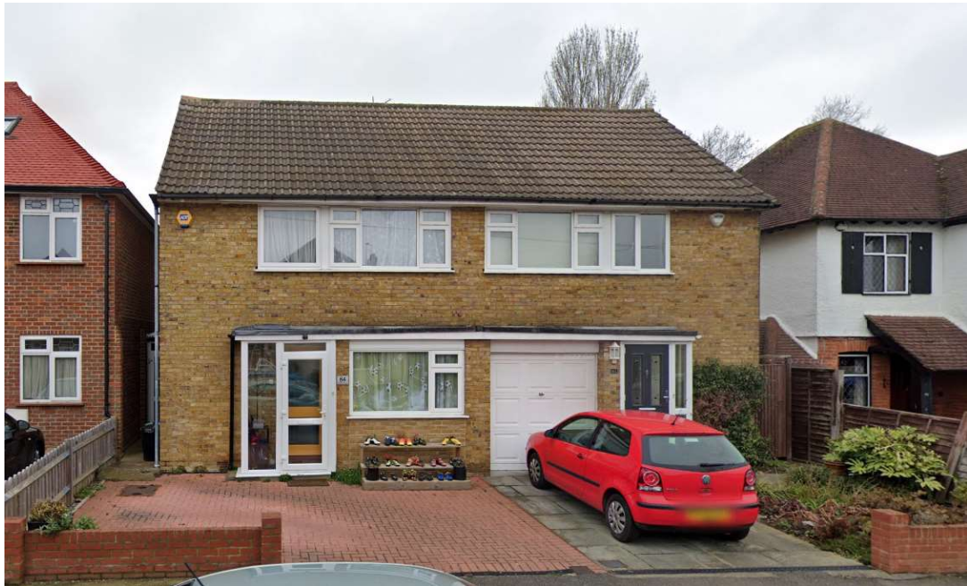
No 64 & 62 Myrtle Avenue – Pair of Two-story semi-detached houses with gable end.
