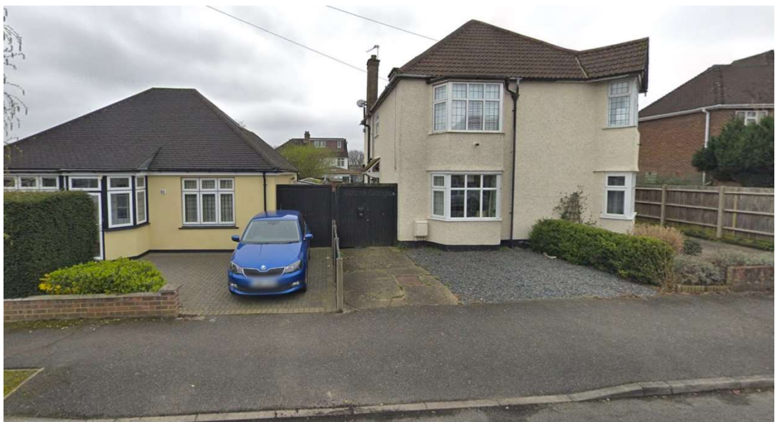
No 53 Myrtle Avenue – Detached bungalow with pitched roof.
