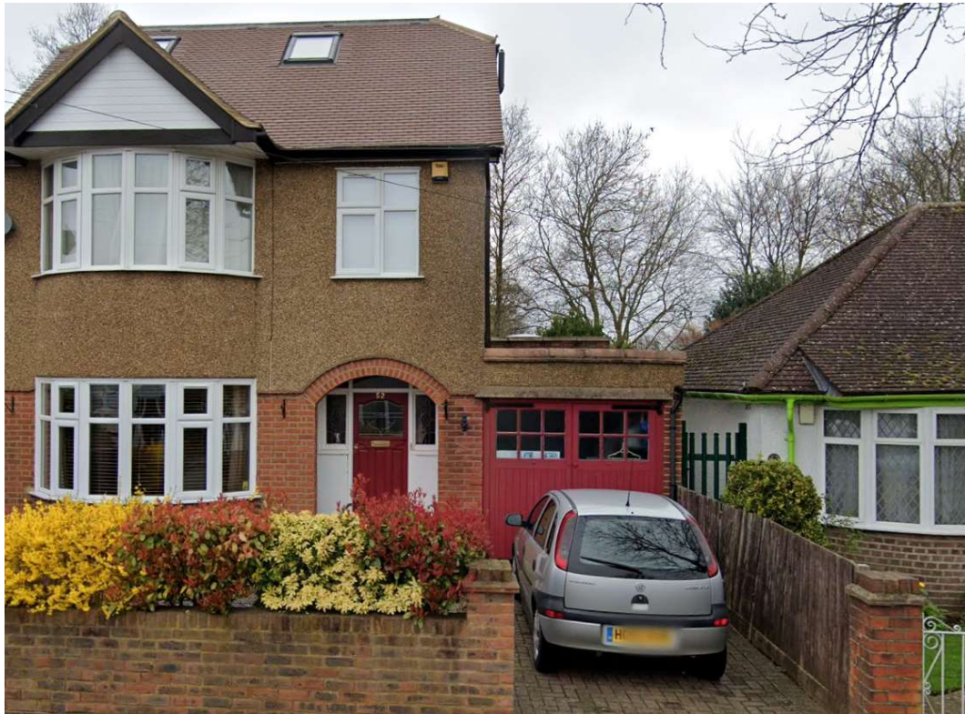
No 52 Myrtle Avenue – Two story detached house with gable roof.
