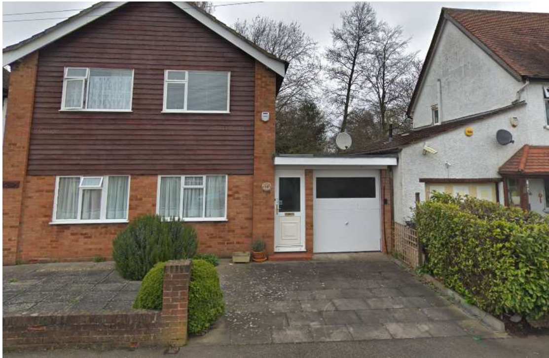
No 58A Myrtle Avenue – Semi-detached two-story house with front gable.
