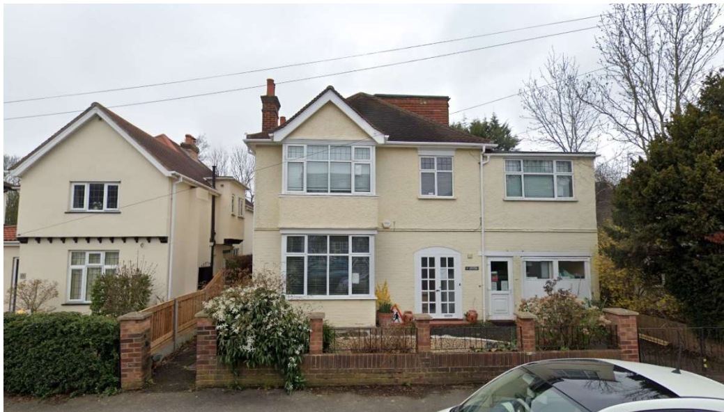
No 16 Myrtle Avenue – Detached two story houses with part pitched and part flat roof.
