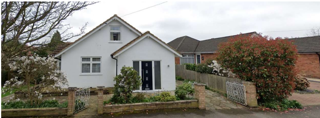
No 45 Myrtle Avenue – Detached bungalow with gable roof.
