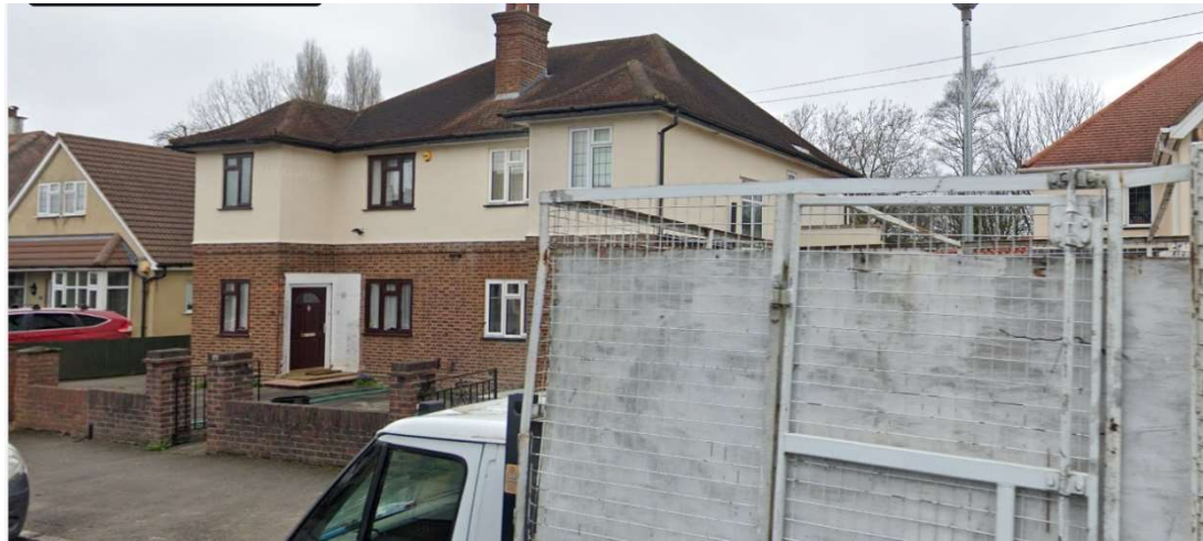
No 20 & 22 Myrtle Avenue – Pair of semi-detached houses with pitched roof.
