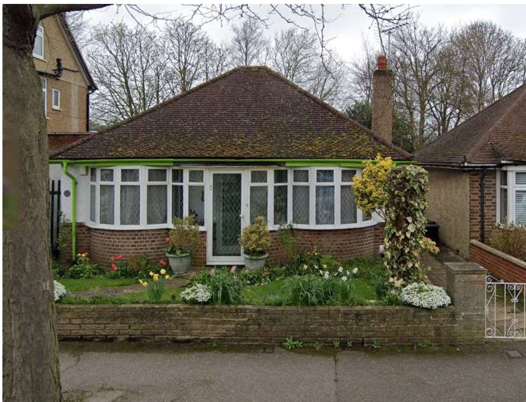
No 50 Myrtle Avenue – Detached bungalow with pitched roof.
