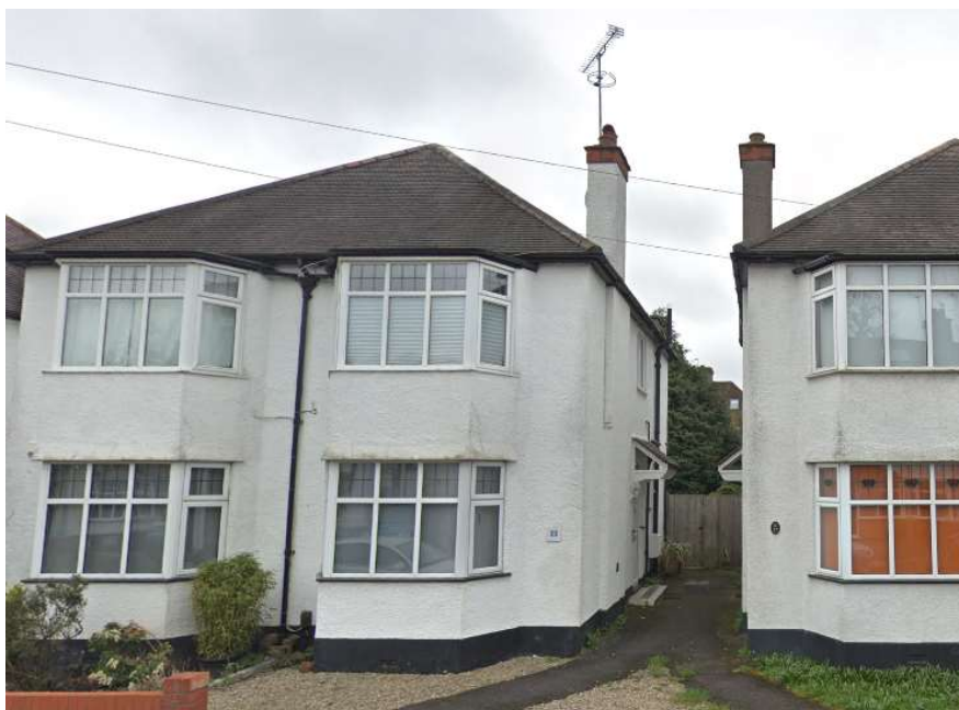
No 23 & 25 Myrtle Avenue – Pair of semi-detached houses with pitched roof.
