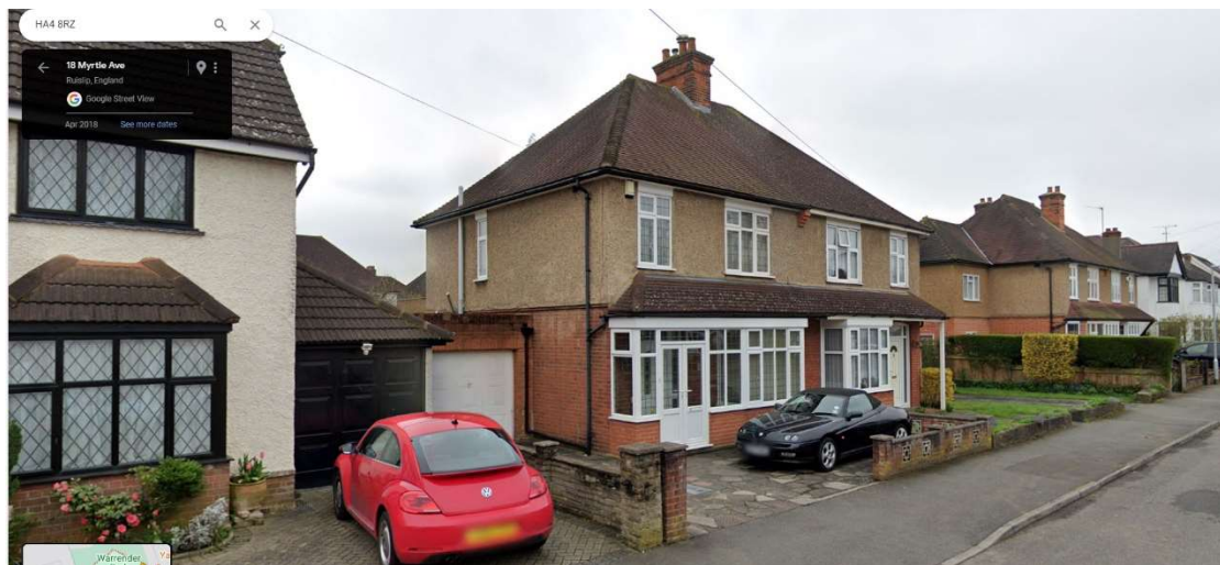
No 13 & 15 Myrtle Avenue – Pair of semi-detached houses with pitched roof.
