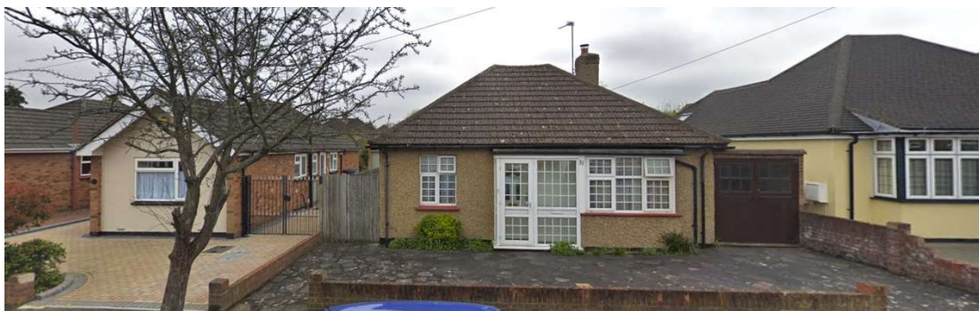
No 51 Myrtle Avenue – Detached bungalow with pitched roof.
