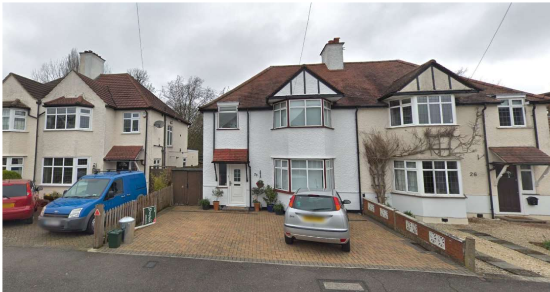
No 26 & 28 Myrtle Avenue – Pair of semi-detached houses with pitched roof.
