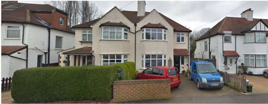
No 30 & 32 Myrtle Avenue – Pair of semi-detached houses with pitched roof.
