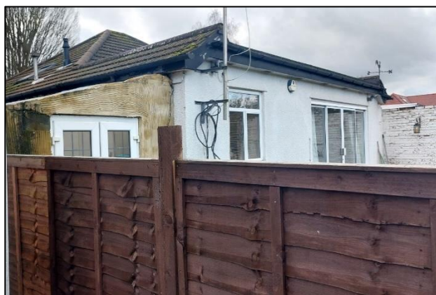
Rear Elevation of No. 44
