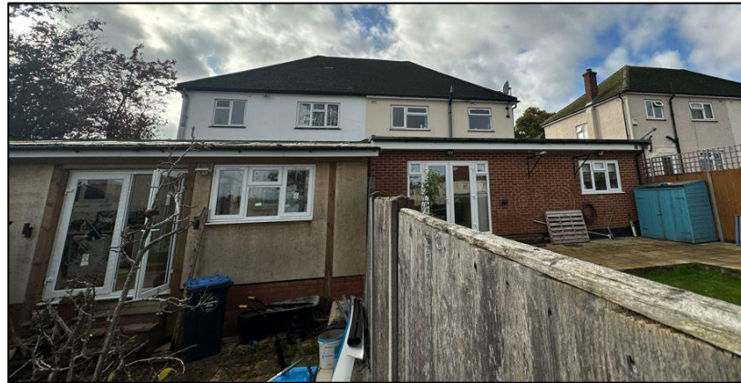
Rear Extensions at Nos. 2 and 4 Rochester Road
