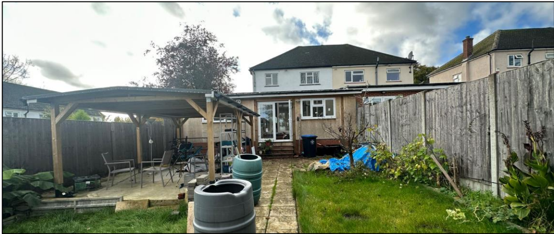
Rear elevation of No. 2 Rochester Road
