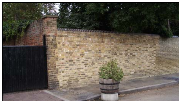
Wall to the west of Summerhouse Lane
