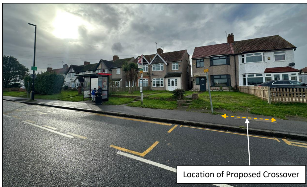
Bus Stop Cage to the South of the Proposed Crossover
