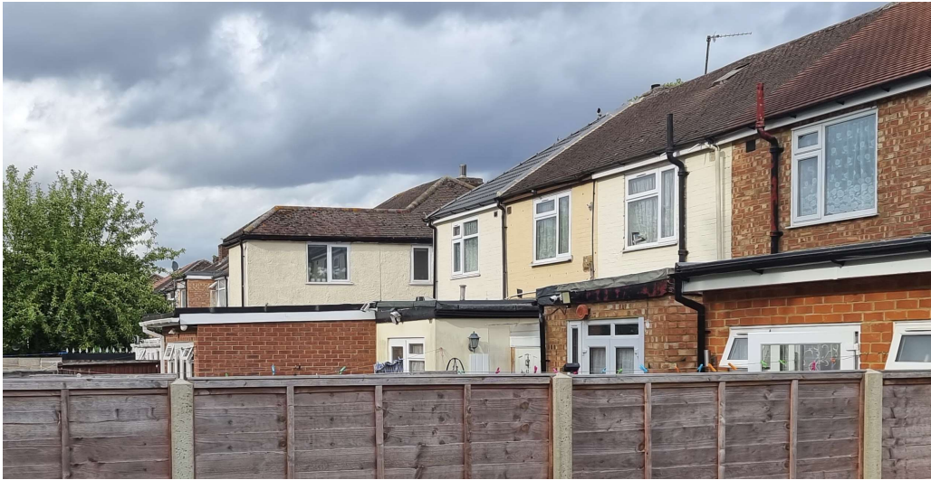
Larger single story extension similar to appeal site along the Fairholme Crescent.
