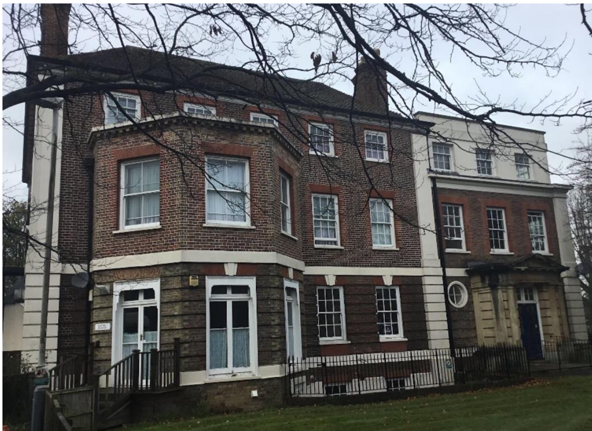
Plate 1 : East elevation of Cowley House
