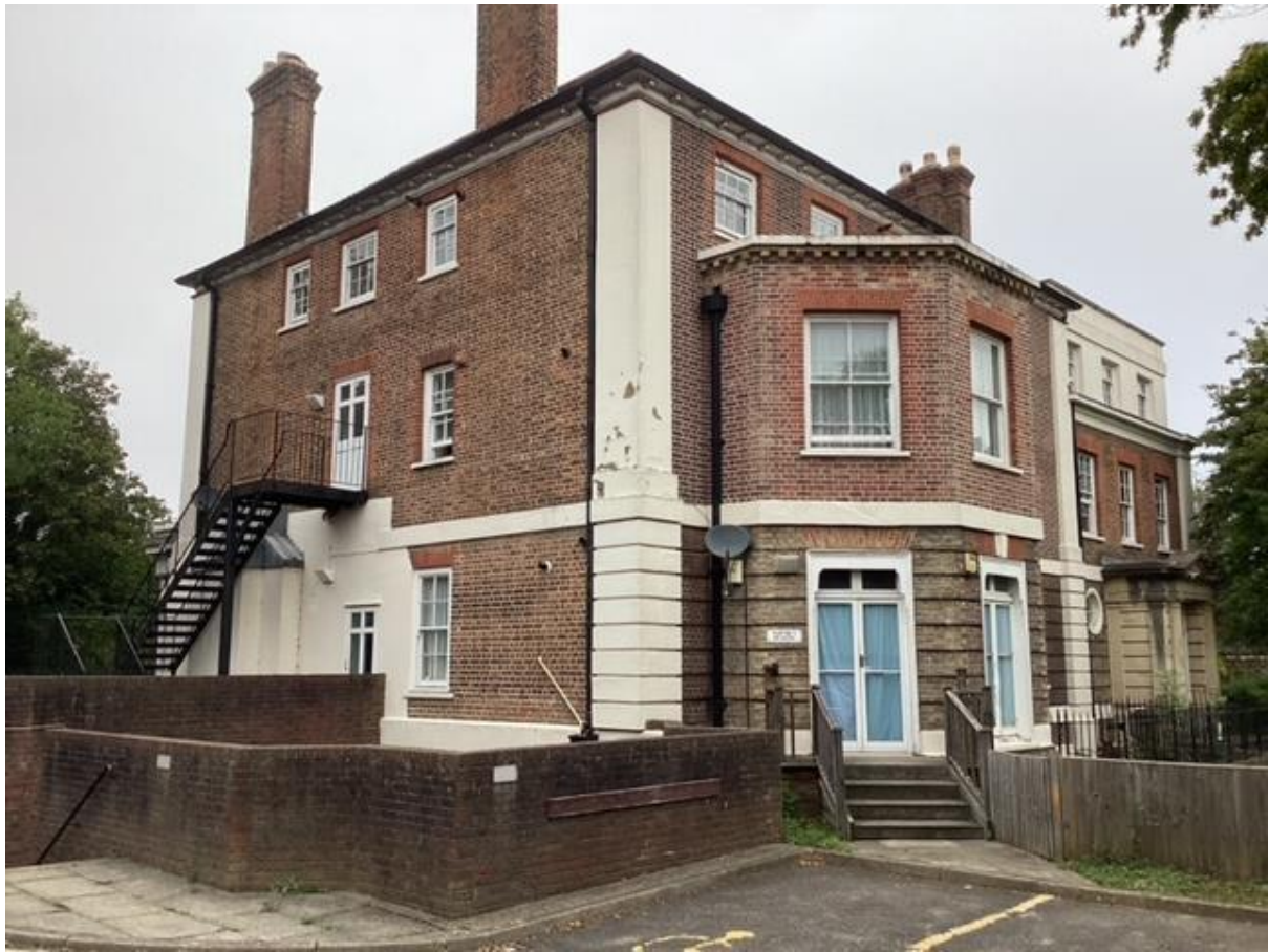
Plate 3: South eastern corner of Cowley House
