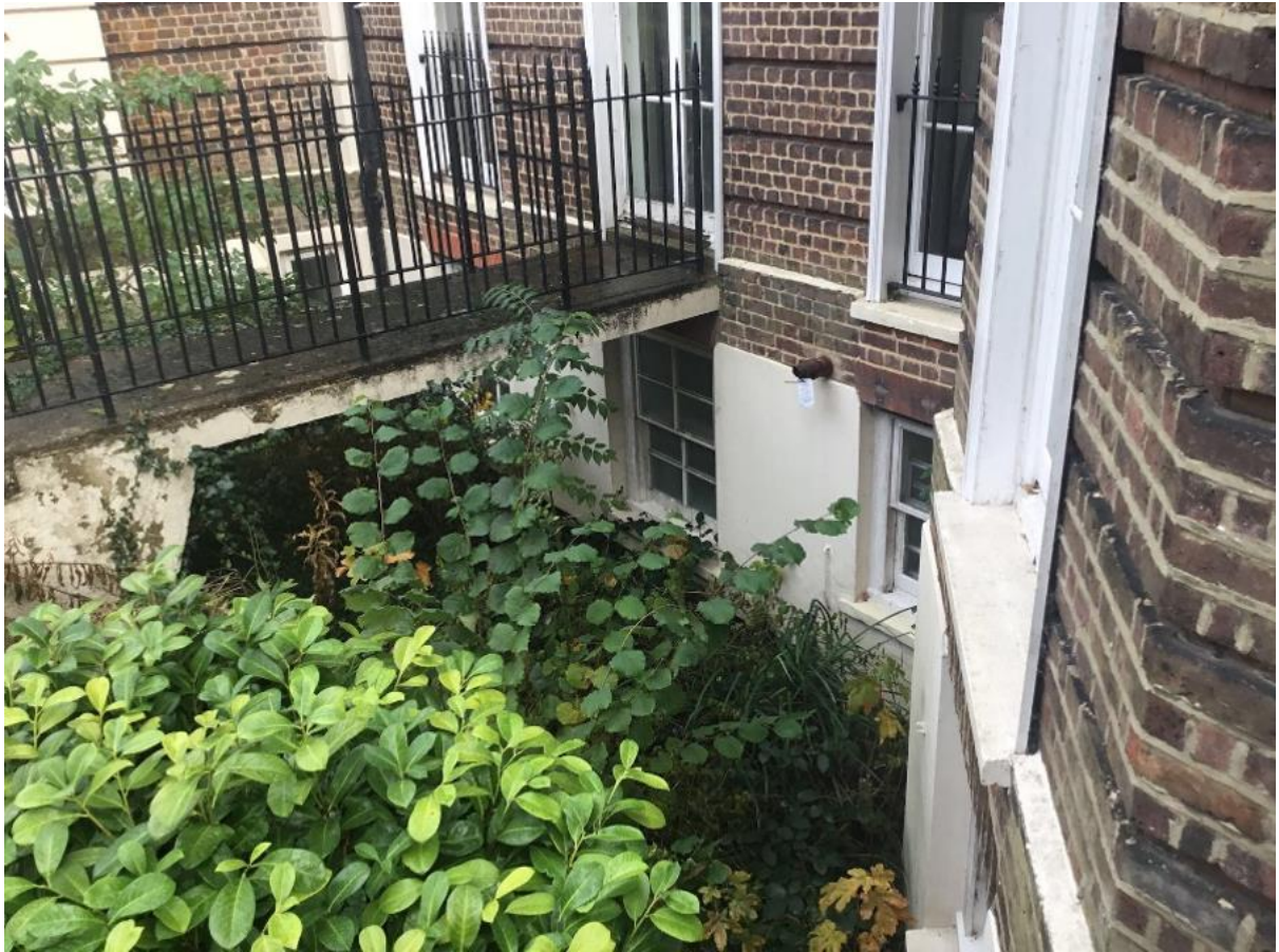
Plate 2: Basement level of west facing elevation
