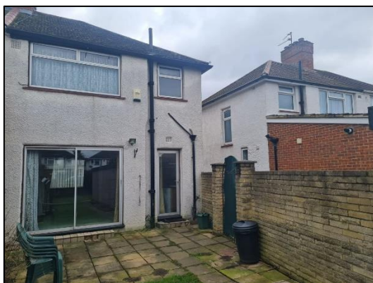
Garden Wall and Gate
