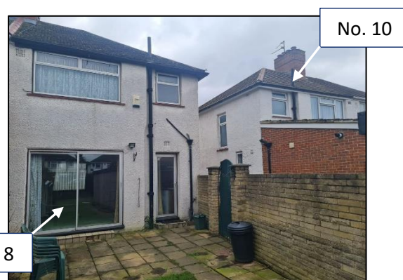
Rear Extension at No. 10 Phelps Way
