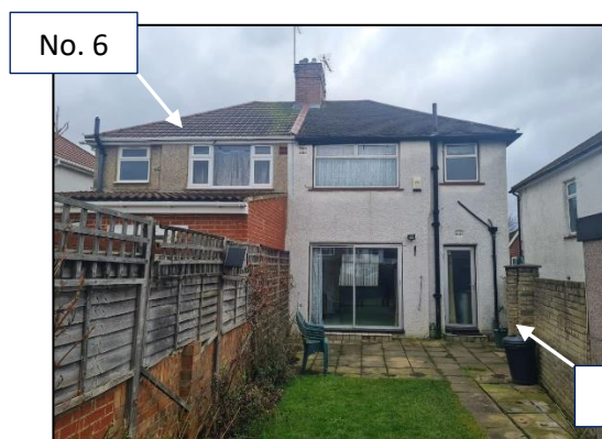
Rear Extension at No. 6 Phelps Way
