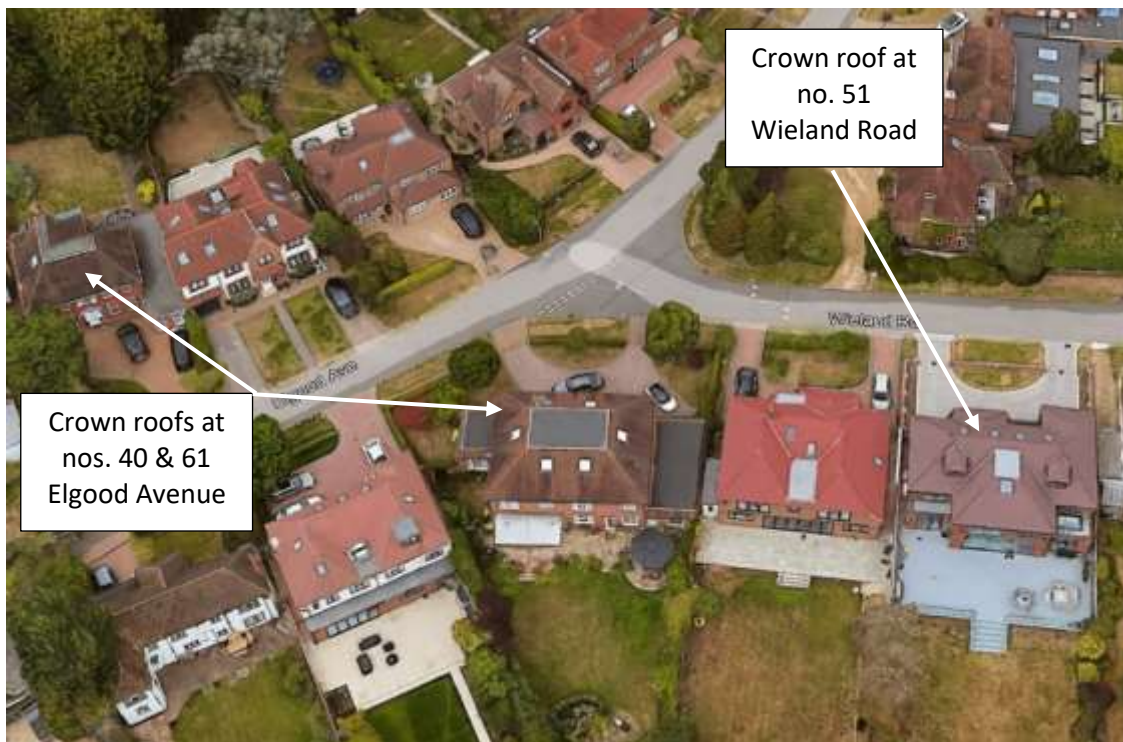
Crown Roofs on the Gatehill Farm Estate
