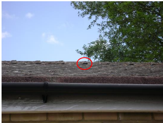
Photograph 3. Raised ridge tile with bat roost potential
