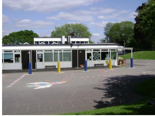
Photograph 2. Example of building on site
