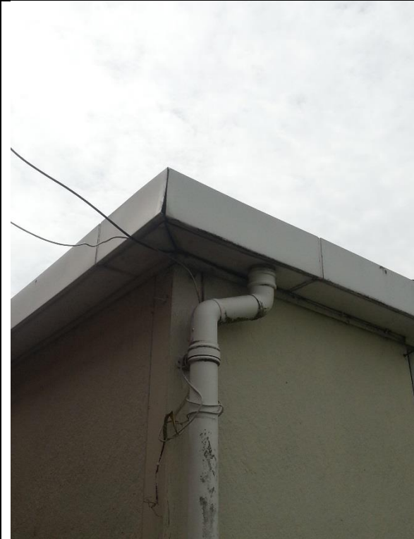
Photograph 15. TN5- Gap providing access to metal soffits..
