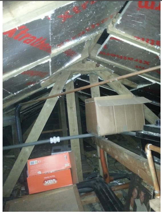
Photograph 2. B1 – internal loft view
