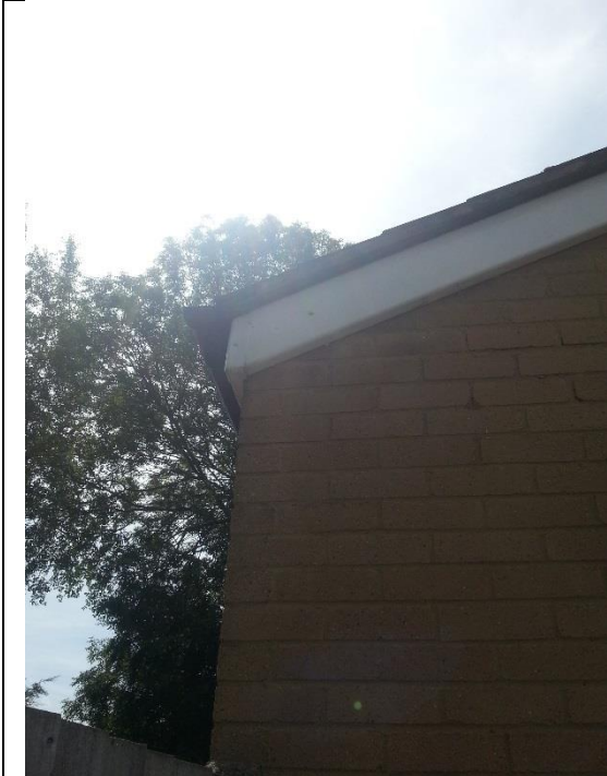
Photograph 11. TN1- Hole in cement underneath tile next to drain pipe.
