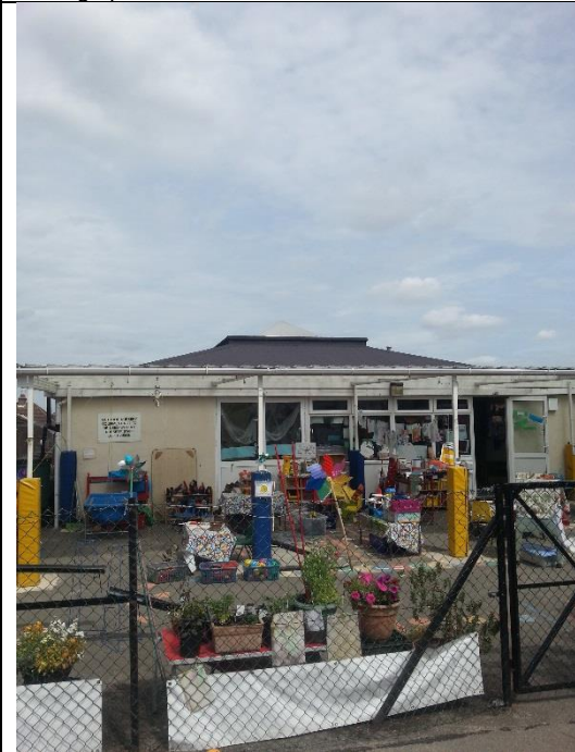
Photograph 7. B7 – south-eastern aspect.
