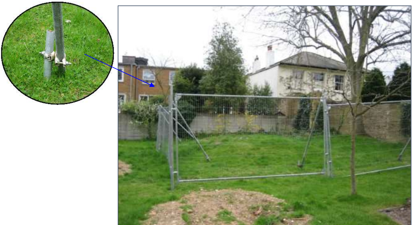
Figure 1 Example of welded mesh barriers in use
