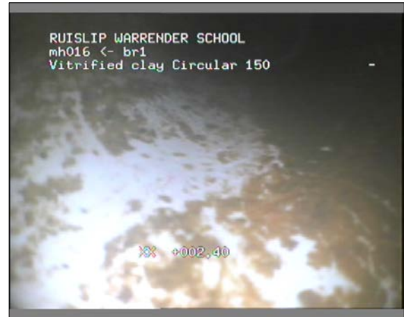
Photo: 58_58_219_A.jpg 2.4m, Finish node type, major connection without manhole reference number: br1
