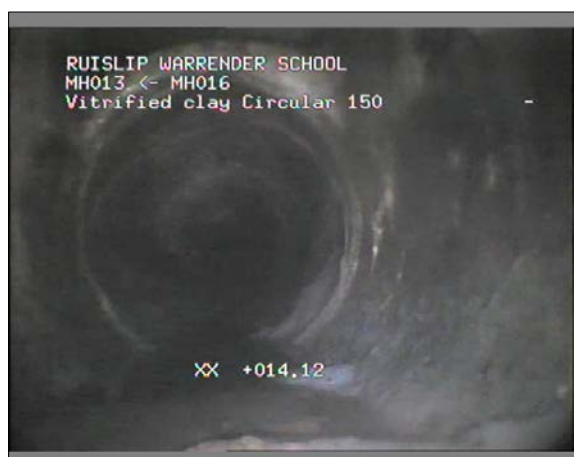
Photo: 45_45_174_A.jpg 14.12m, Finish node type, manhole reference number: MH016
