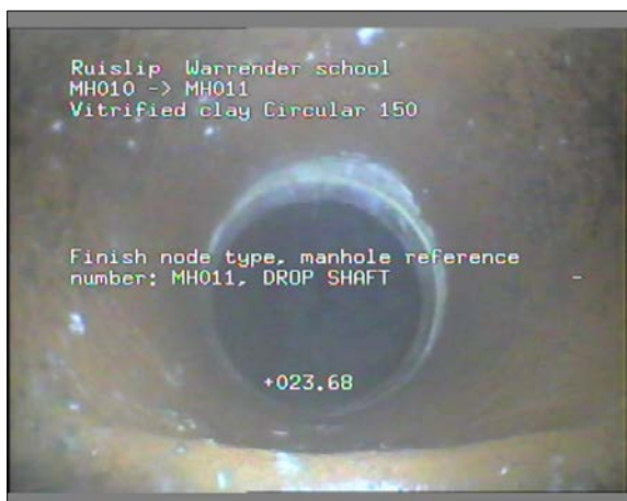
Photo: 35_35_137_A.JPG 23.68m, Finish node type, manhole reference number: MH011
