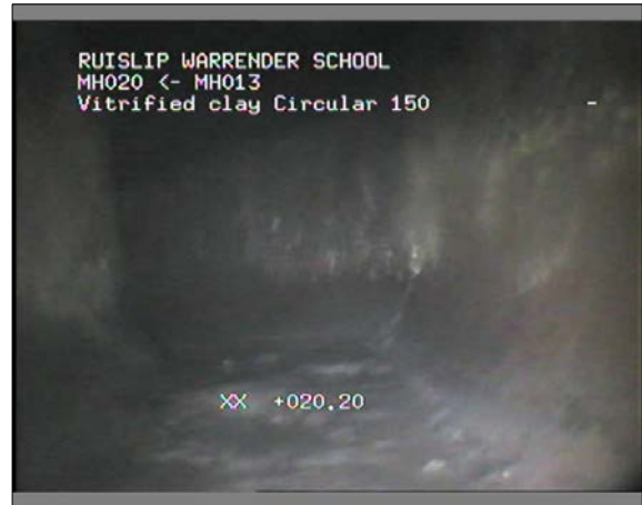
Photo: 44_44_170_A.jpg 20.2m, Finish node type, manhole reference number: MH013
