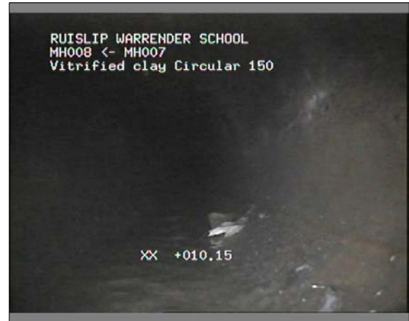
Photo: 36_36_142_A.jpg 10.15m, Finish node type, manhole reference number: MH007
