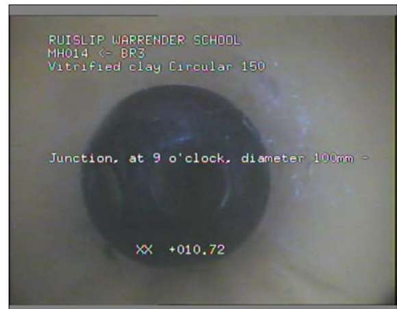
Photo: 50_50_193_A.jpg 10.72m, Junction, at 9 o'clock, diameter 100mm
