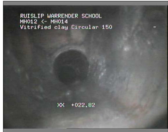
Photo: 41_41_160_A.jpg 22.82m, Finish node type, manhole reference number: MH014
