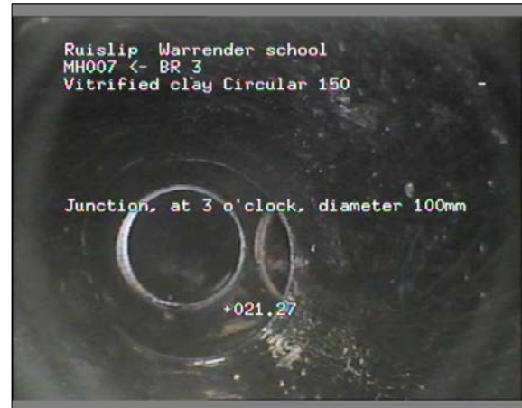
Photo: 20_20_82_A.JPG 21.27m, Junction, at 3 o'clock, diameter 100mm
