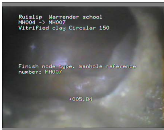
Photo: 13_13_52_A.JPG 5.84m, Finish node type, manhole reference number: MH007
