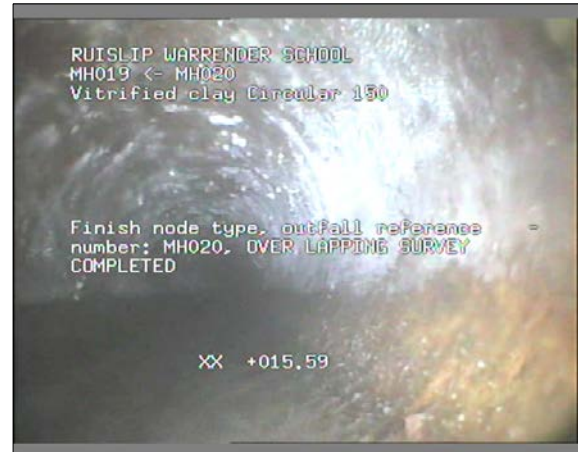
Photo: 56_56_213_A.jpg 15.64m, Finish node type, outfall reference number: MH020
