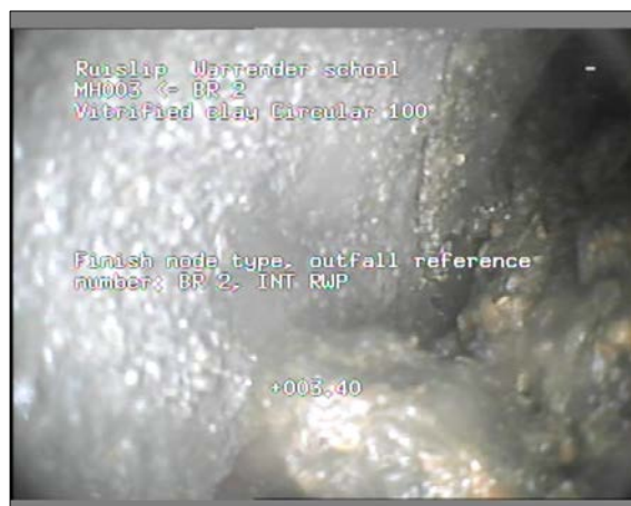
Photo: 8_8_33_A.JPG 3.4m, Finish node type, outfall reference number: BR 2
