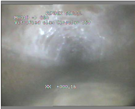
Photo: 57_57_214_A.jpg 0.07m, Start node type, manhole, reference number : MH019
