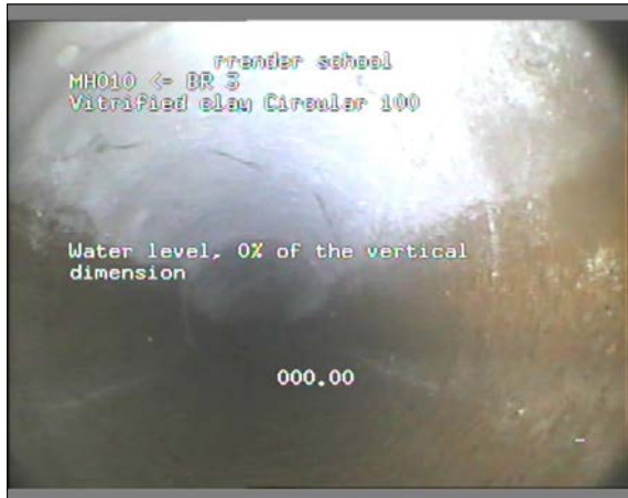
Photo: 31_31_121_A.JPG 0m, Start node type, manhole, reference number : MH010
