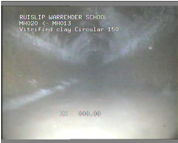
Photo: 44_44_169_A.jpg 0m, Start node type, manhole, reference number : MH020
