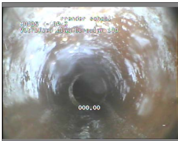
Photo: 16_16_62_A.JPG 0.19m, Start node type, manhole, reference number : MH005
