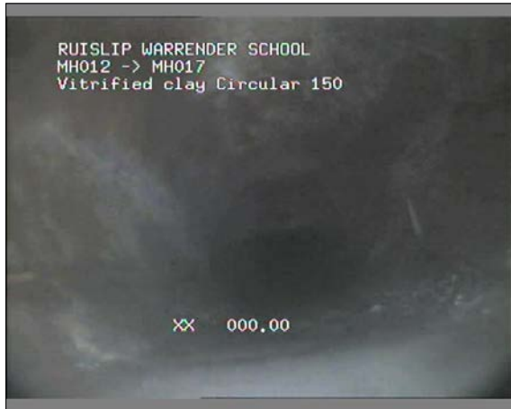
Photo: 39_39_153_A.jpg 0m, Start node type, manhole, reference number : MH012
