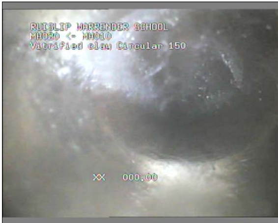
Photo: 43_43_166_A.jpg 0m, Start node type, manhole, reference number : MH020
