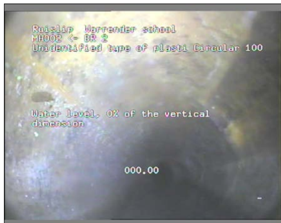
Photo: 4_4_10_A.JPG 0m, Start node type, manhole, reference number : MH002
