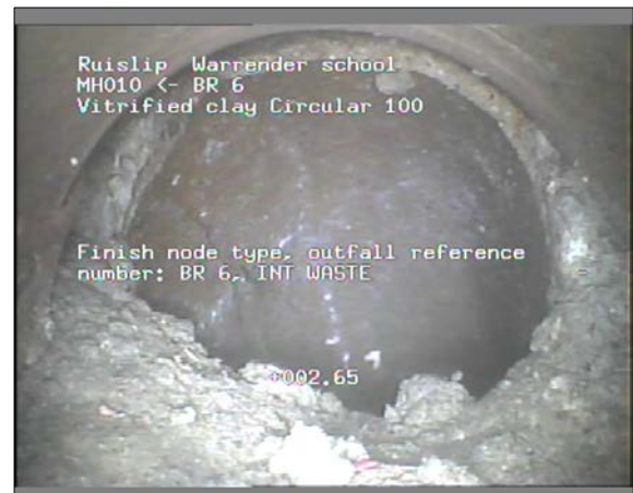
Photo: 34_34_134_A.JPG 2.65m, Finish node type, outfall reference number: BR 6
