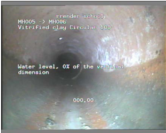
Photo: 17_17_66_A.JPG 0m, Start node type, manhole, reference number : MH005
