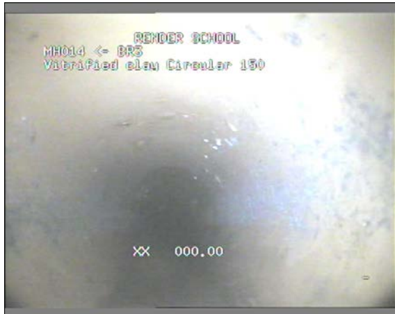
Photo: 50_50_190_A.jpg 0m, Start node type, manhole, reference number : MH014
