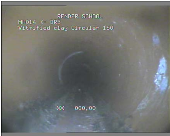
Photo: 52_52_200_A.jpg 0m, Start node type, manhole, reference number : MH014
