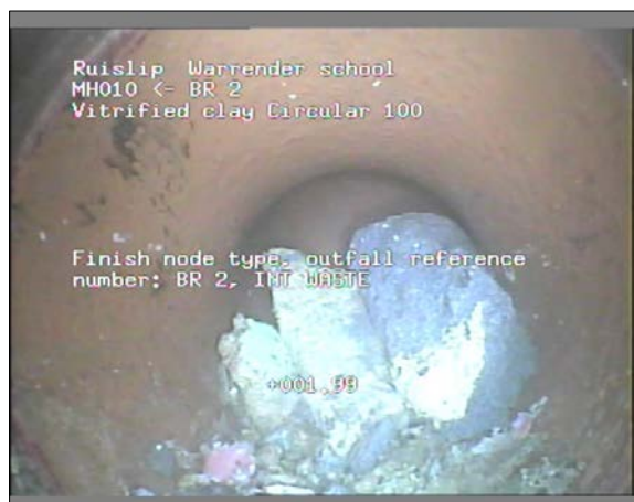
Photo: 30_30_120_A.JPG 1.99m, Finish node type, outfall reference number: BR 2
