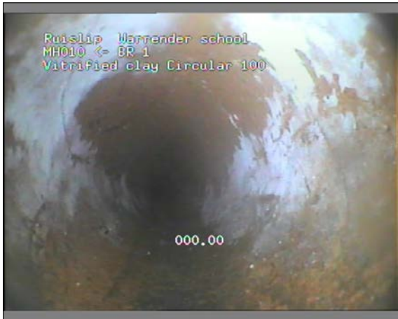
Photo: 29_29_115_A.JPG 0m, Start node type, manhole, reference number : MH010
