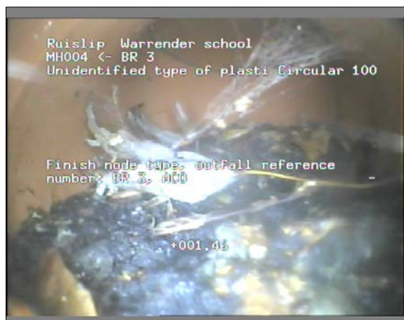
Photo: 12_12_47_A.JPG 1.46m, Finish node type, outfall reference number: BR 3
