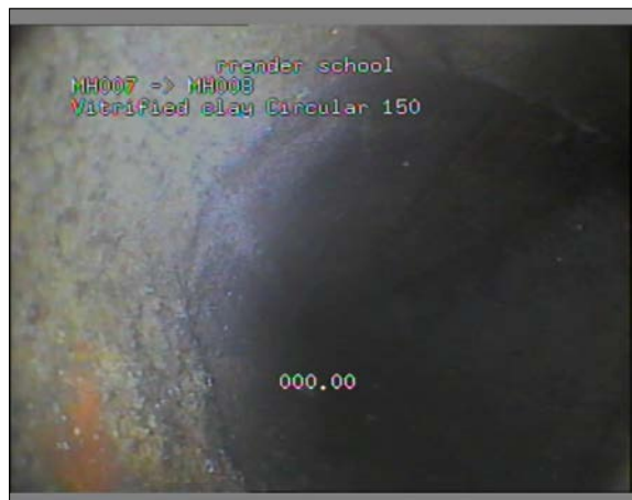
Photo: 21_21_84_A.JPG -0.4m, Start node type, manhole, reference number : MH007
