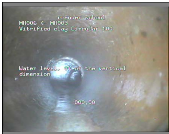
Photo: 22_22_89_A.JPG 0m, Start node type, manhole, reference number : MH006
