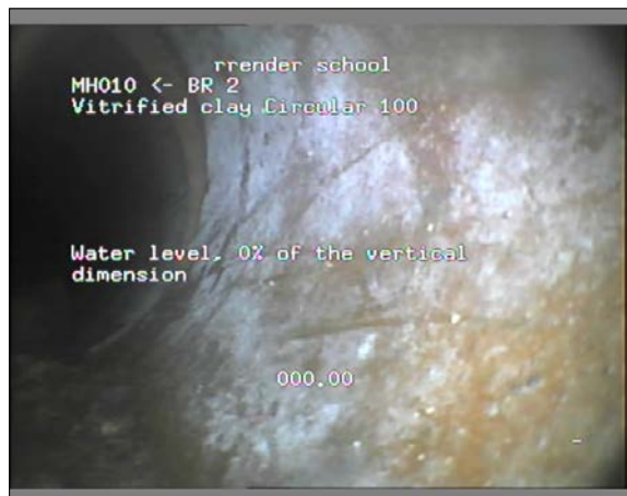
Photo: 30_30_118_A.JPG 0m, Start node type, manhole, reference number : MH010
