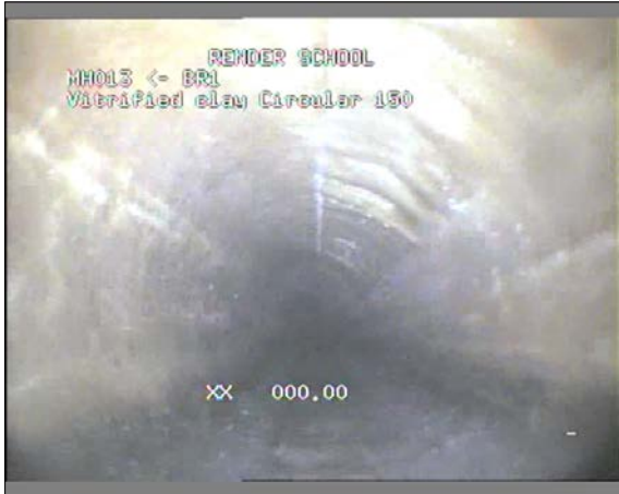
Photo: 47_47_179_A.jpg 0m, Start node type, manhole, reference number : MH013
