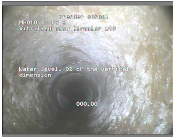
Photo: 34_34_131_A.JPG 0m, Start node type, manhole, reference number : MH010
