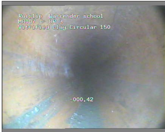
Photo: 20_20_77_A.JPG 0m, Start node type, manhole, reference number : MH007
