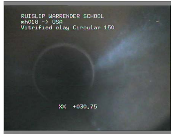
Photo: 55_55_210_A.jpg 30.76m, Finish node type, outfall reference number: OSA
