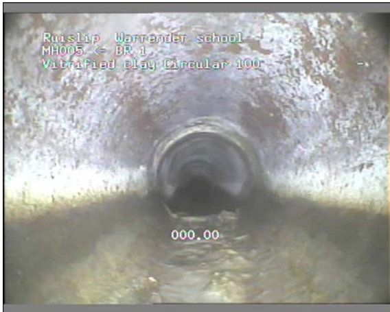
Photo: 14_14_53_A.JPG 0m, Start node type, manhole, reference number : MH005
