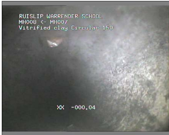
Photo: 36_36_139_A.jpg 0m, Start node type, manhole, reference number : MH008
