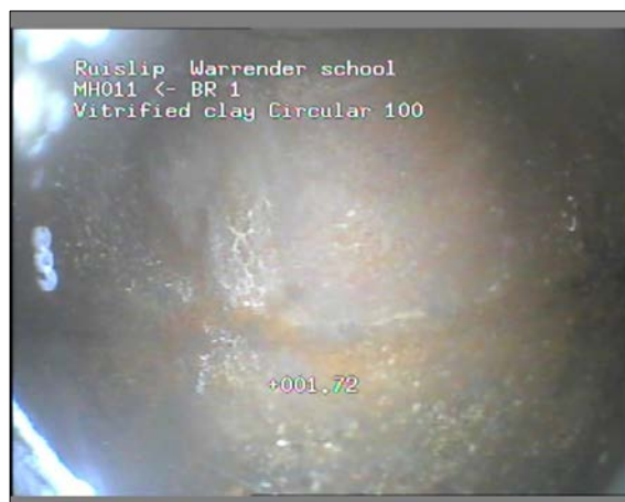
Photo: 27_27_111_A.JPG 1.72m, Finish node type, outfall reference number: BR 1
