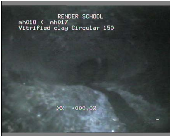
Photo: 54_54_206_A.jpg 0m, Start node type, manhole, reference number : mh018
