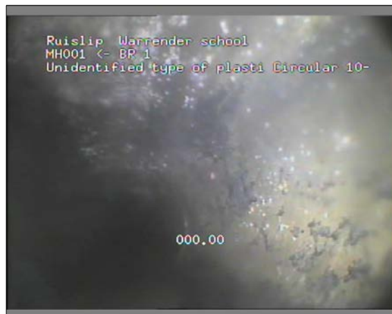
Photo: 6_6_21_A.JPG 1.08m, Start node type, manhole, reference number : MH001
