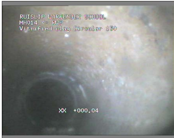
Photo: 42_42_162_A.jpg 0m, Start node type, manhole, reference number : MH014
