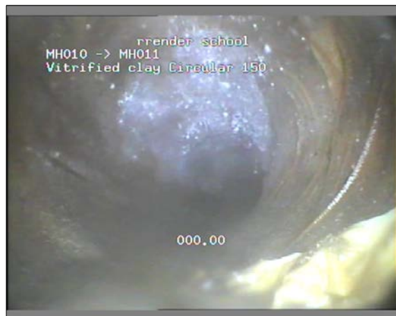
Photo: 35_35_135_A.JPG -0.56m, Start node type, manhole, reference number : MH010
