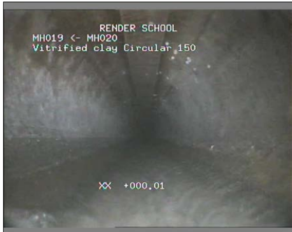
Photo: 56_56_212_A.jpg 0m, Start node type, manhole, reference number : MH019
