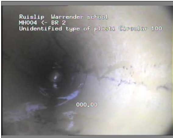
Photo: 11_11_42_A.JPG 0m, Start node type, manhole, reference number : MH004
