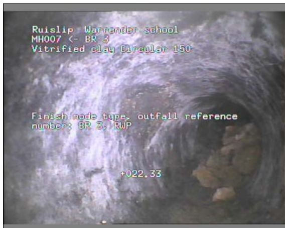
Photo: 20_20_83_A.JPG 22.33m, Finish node type, outfall reference number: BR 3
