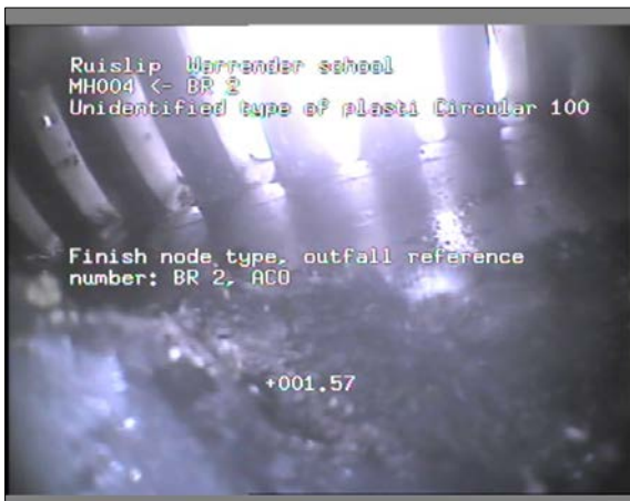
Photo: 11_11_44_A.JPG 1.57m, Finish node type, outfall reference number: BR 2
