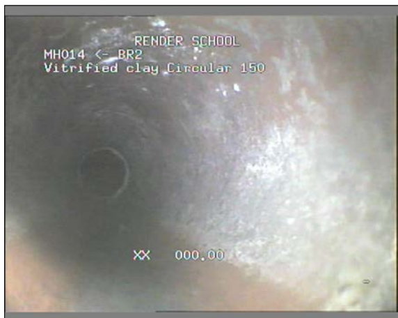
Photo: 49_49_186_A.jpg 0m, Start node type, manhole, reference number : MH014
