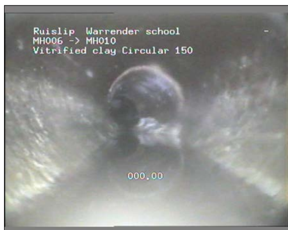
Photo: 26_26_103_A.JPG 0m, Start node type, manhole, reference number : MH006
