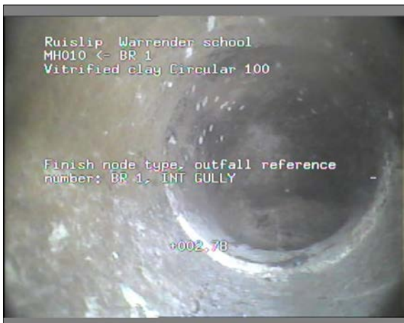
Photo: 29_29_117_A.JPG 2.78m, Finish node type, outfall reference number: BR 1
