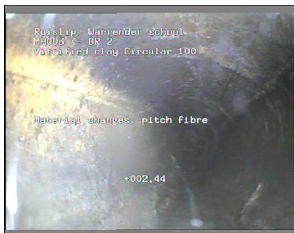
Photo: 8_8_32_A.JPG 2.44m, Material changes, pitch fibre
