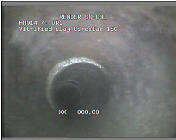
Photo: 48_48_182_A.jpg 0m, Start node type, manhole, reference number : MH014
