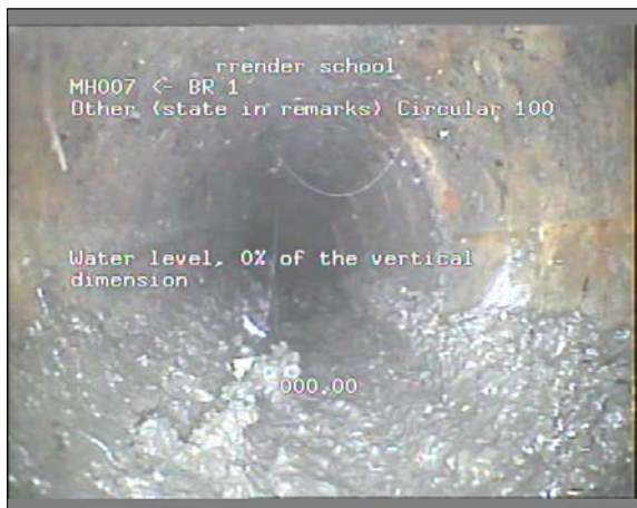
Photo: 18_18_69_A.JPG 0m, Start node type, manhole, reference number : MH007
