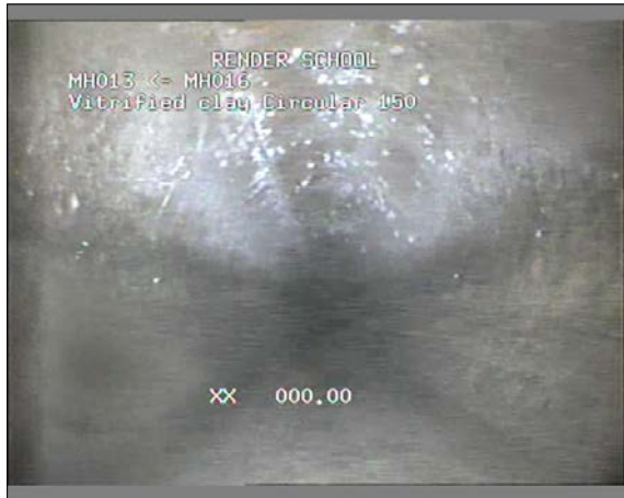
Photo: 45_45_172_A.jpg 0m, Start node type, manhole, reference number : MH013
