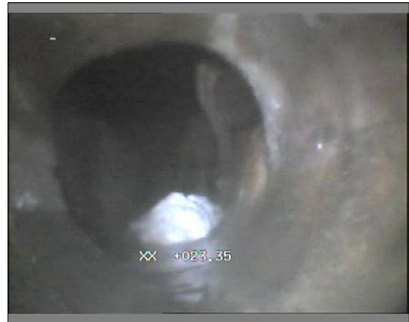
Photo: 43_43_167_A.jpg 23.35m, Finish node type, manhole reference number: MH010
