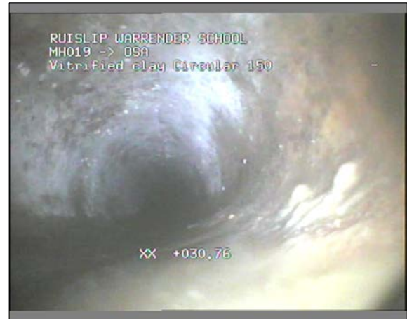
Photo: 57_57_216_A.jpg 30.69m, Finish node type, outfall reference number: OSA
