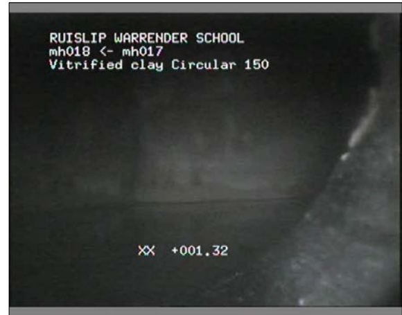
Photo: 54_54_207_A.jpg 1.32m, Finish node type, manhole reference number: mh017
