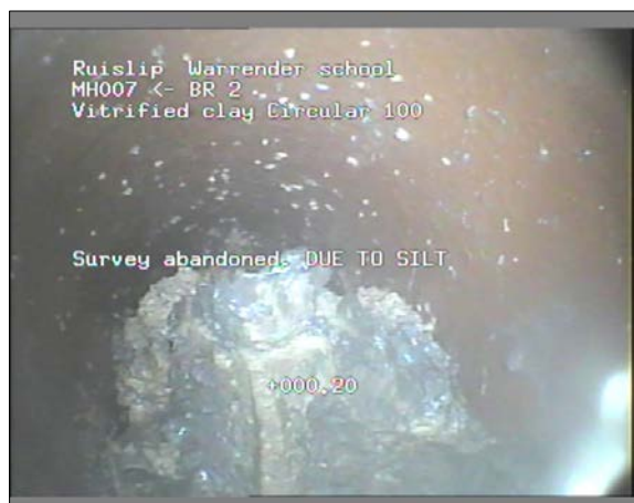
Photo: 19_19_75_A.JPG 0.2m, Settled deposits, fine, 90% cross-sectional area loss
