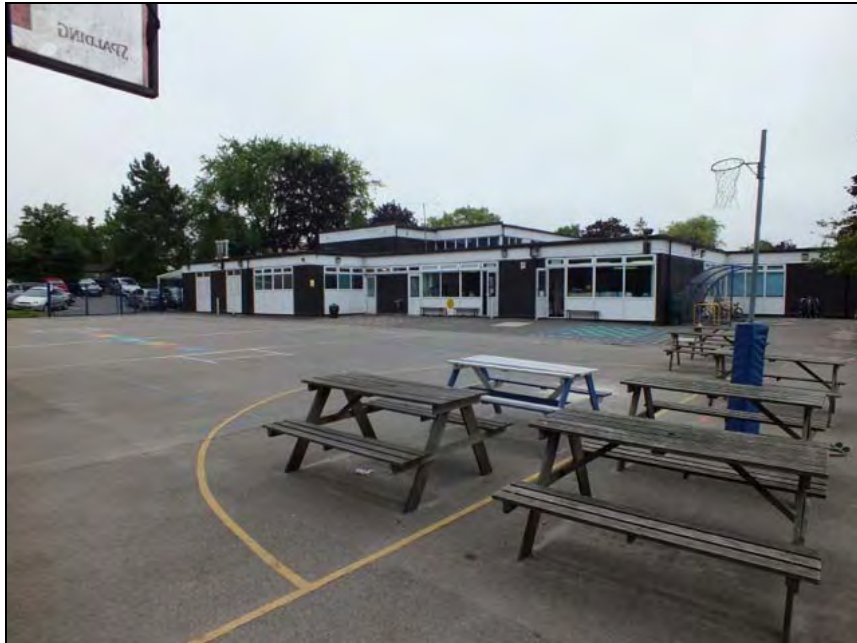
Plate 7: View south across junior playground towards school buildings
