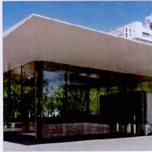
Glazing : Schüco curtain wall system
