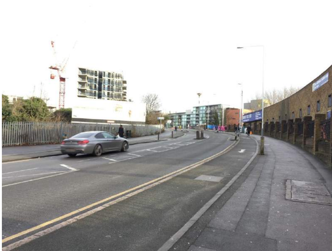
Photo 5 – Southbound off-road cycle lane on Station Road
