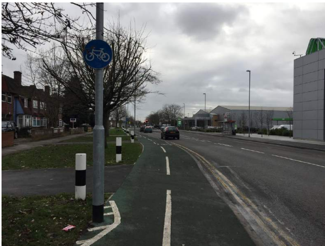
Photo 3 – Station Roads Two-way cycle lane
