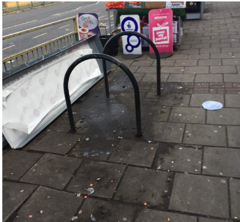
Photo 11 – Sheffield Stands suffering from obstructions, litter and ponding on North Hyde Road (CP3)
