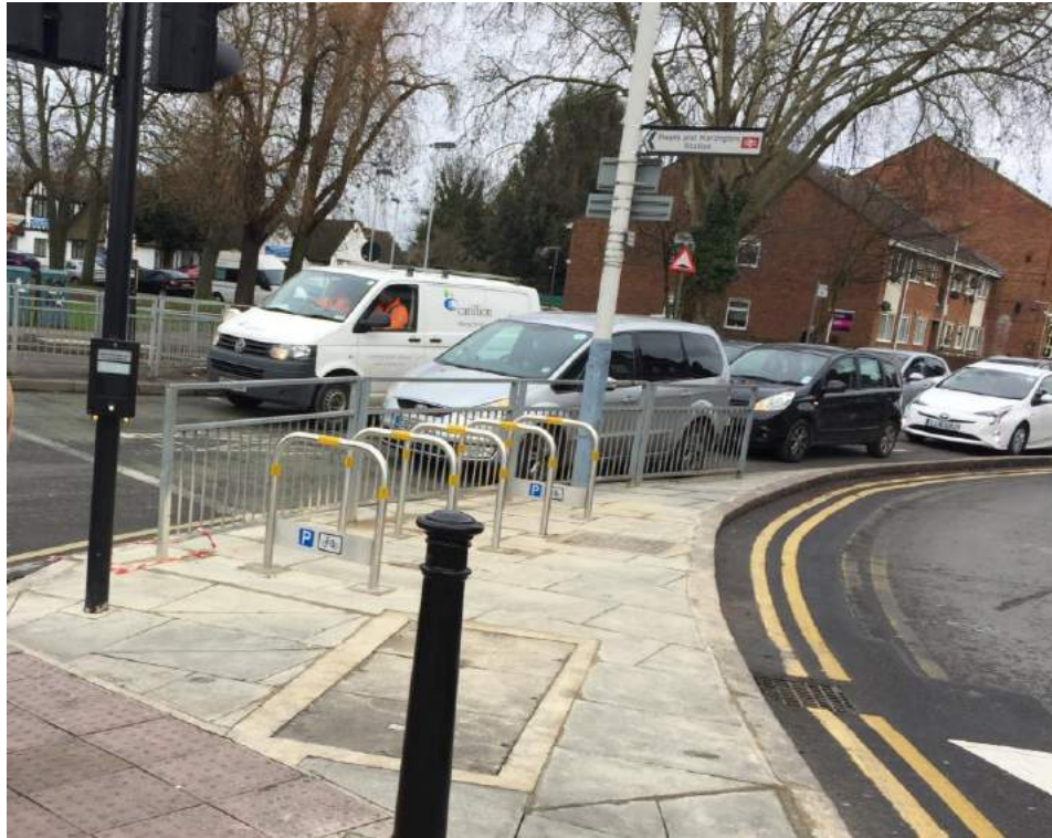
Photo 11 – Sheffield Stands suffering from obstructions, litter and ponding on North Hyde Road (CP3)
