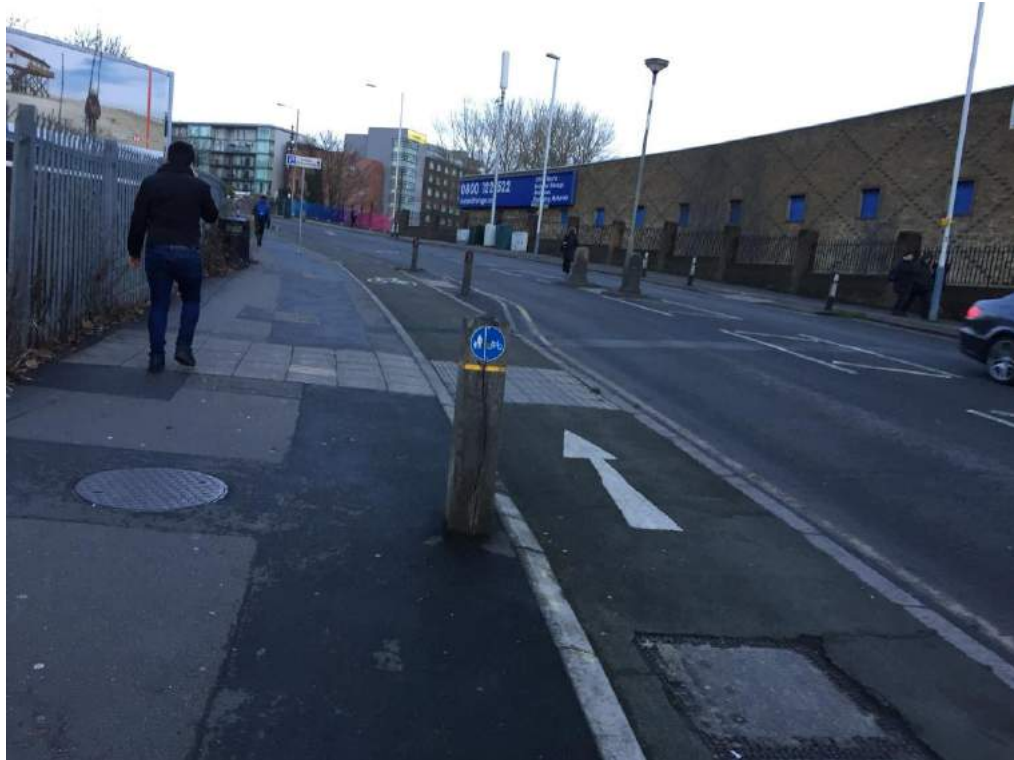
Photo 4 – Northbound off-road cycle lane on Station Road
