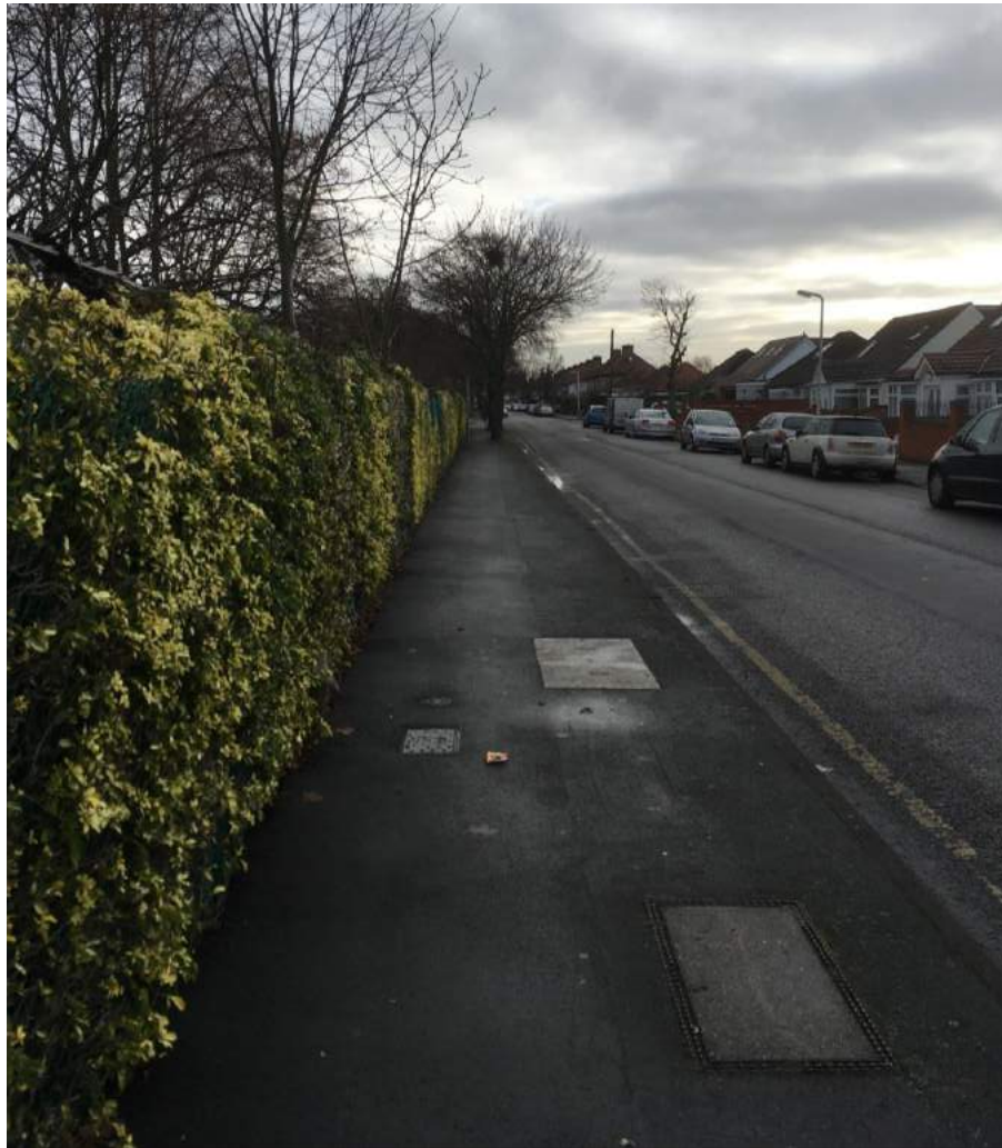
Photo 1 – North Western side of Footway, Nestle Avenue
