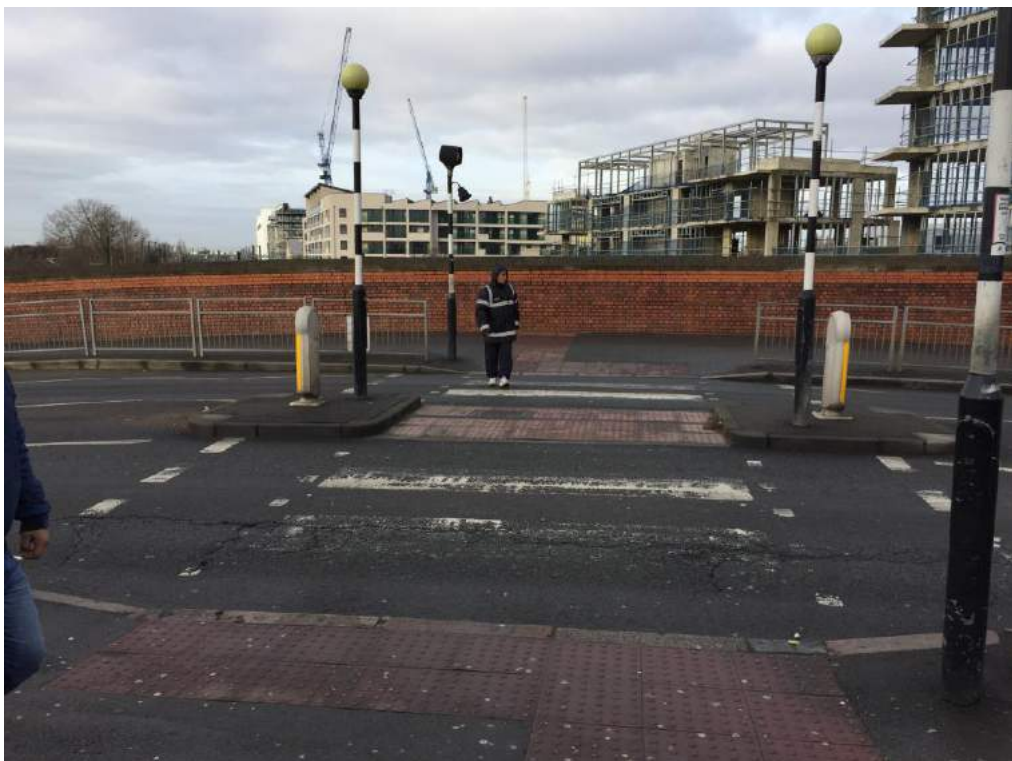
Photo 11 – Station Road - Zebra Crossing (C2)
