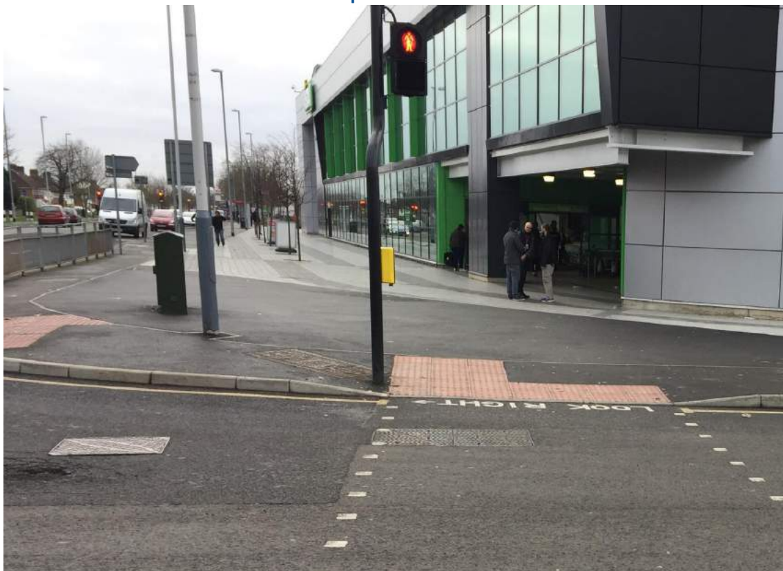
Photo 6 – Improved pedestrian footpath and pedestrian crossing outside the new ASDA supermarket
