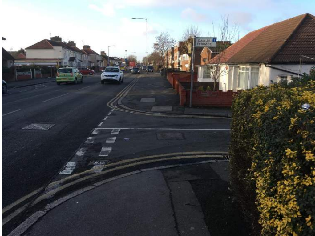
Photo 14 – Lack of tactile at the North Hyde / Dallas Terrace junction
