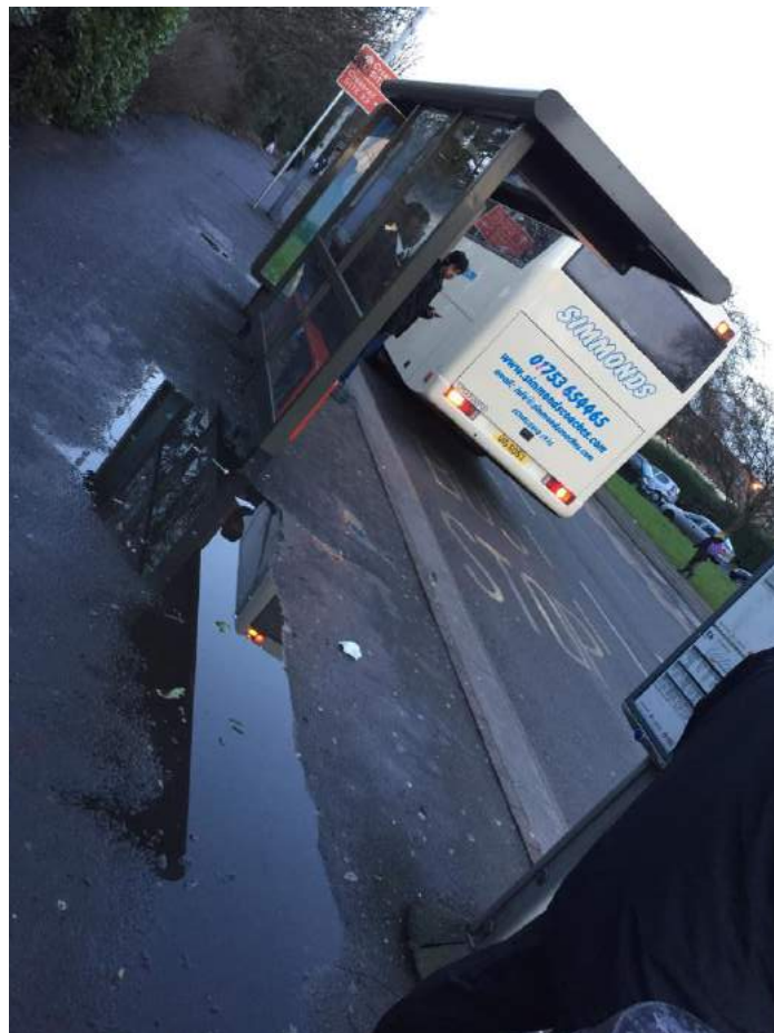
Photo 15 - Sheltered bus stop located to the north of the Station Road / North Hyde Road Junction
