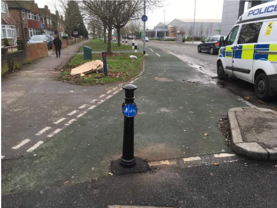
Photo 5 – Station Road eastern side, with segregated pedestrian footway and cycle lane
