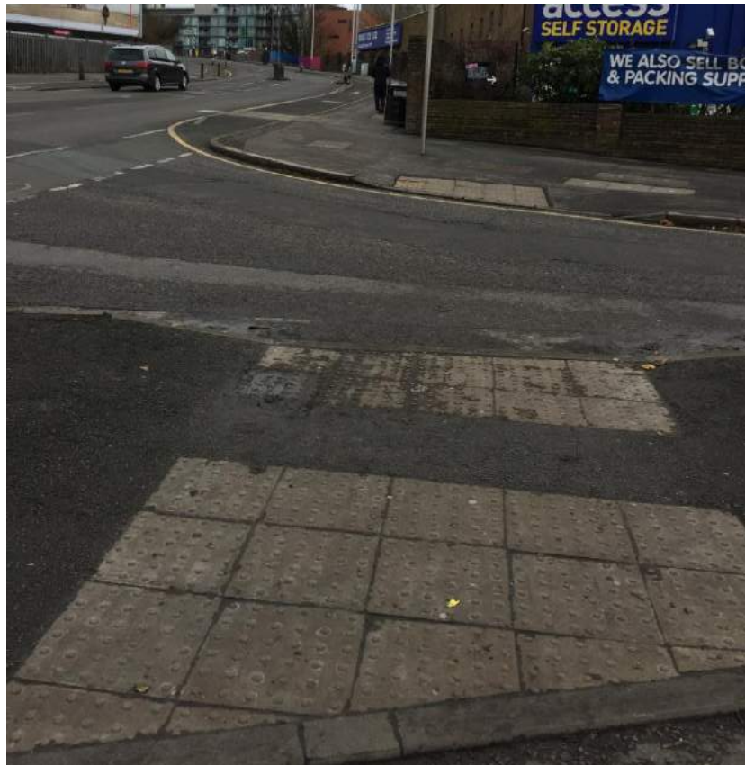
Photo 10 – Junction of Nestle Avenue / Station Road – Refuge Island Crossing (C1)
