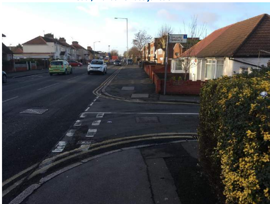
Photo 4 – North Hyde Road footway widths and lack of tactile information on the North Hyde Road / Dallas Terrace junction
