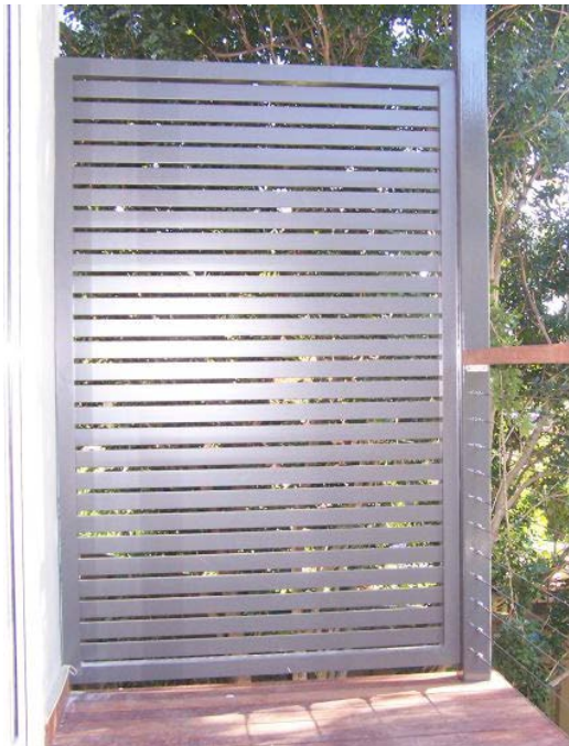
Figure 20: Example of balcony screens
