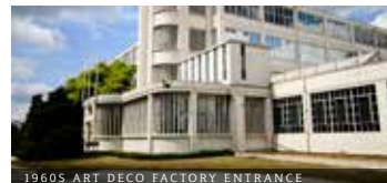
1960S ART DECO FACTORY ENTRANCE
