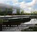
FIG. 4. VIEW OF THE COMMERCIAL OFFICES OVERLOOKING THE CANAL
