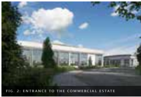
FIG. 2. ENTRANCE TO THE COMMERCIAL ESTATE
