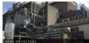
REAR OF FACTORY
