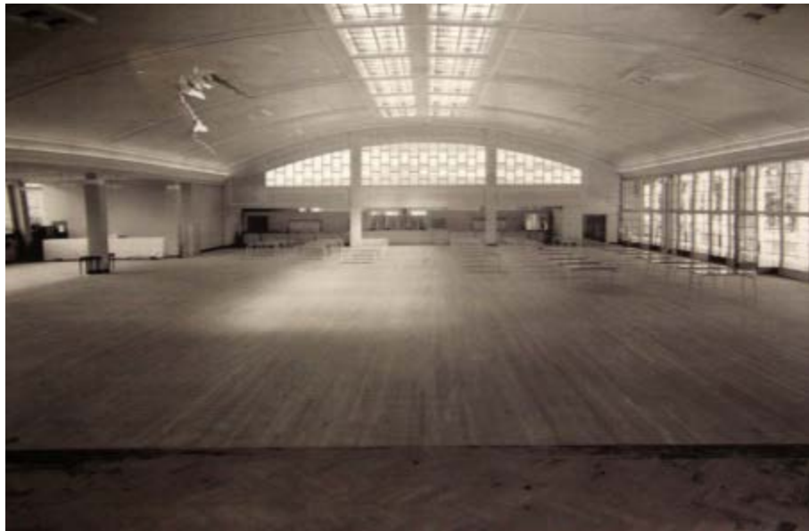
Figure 3.28: Undated image of the interior of the canteen looking north (Hillingdon Local Archives)
