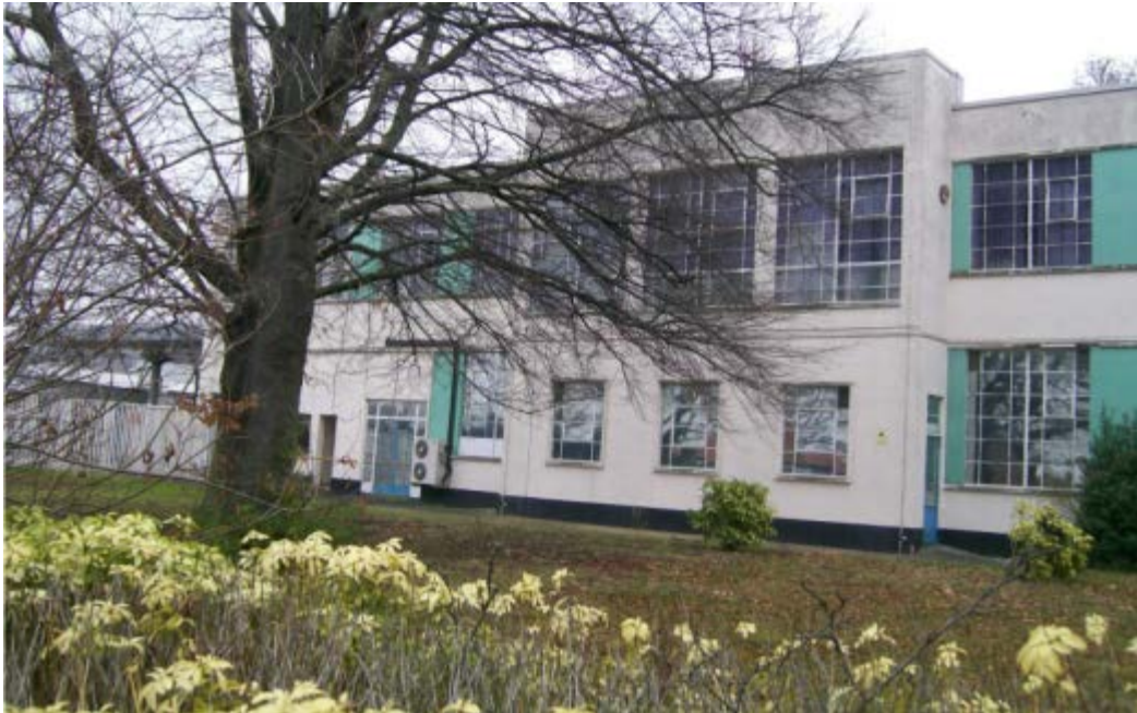
Figure 3.26: View of the south elevation of the former canteen building
