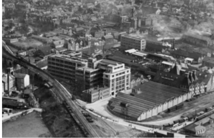
Figure 3.23: The former Tilling-Stevens Factory, 1917 by Wallis Gilbert & Partners in collaboration with Truscon (aerial photograph dated 1921, Britain from Above)
