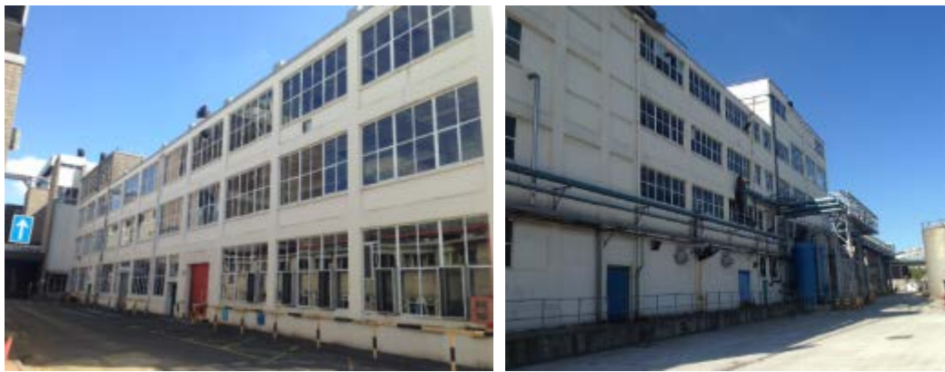
Figure 3.22: View of the west elevation of the Truscon factory
