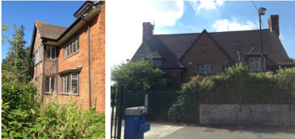
Figure 3.32: (Left) View of the timber framed two storey projecting gable to the front south elevation and (right) the north elevation of the former lodge
