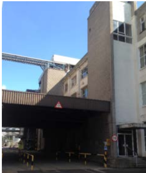
Figure 3.24: View of the west elevation with remains of the original 1914 Sandow building partially visible
