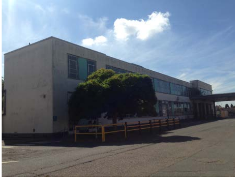
Figure 3.17: View of the west elevation of the former canteen
