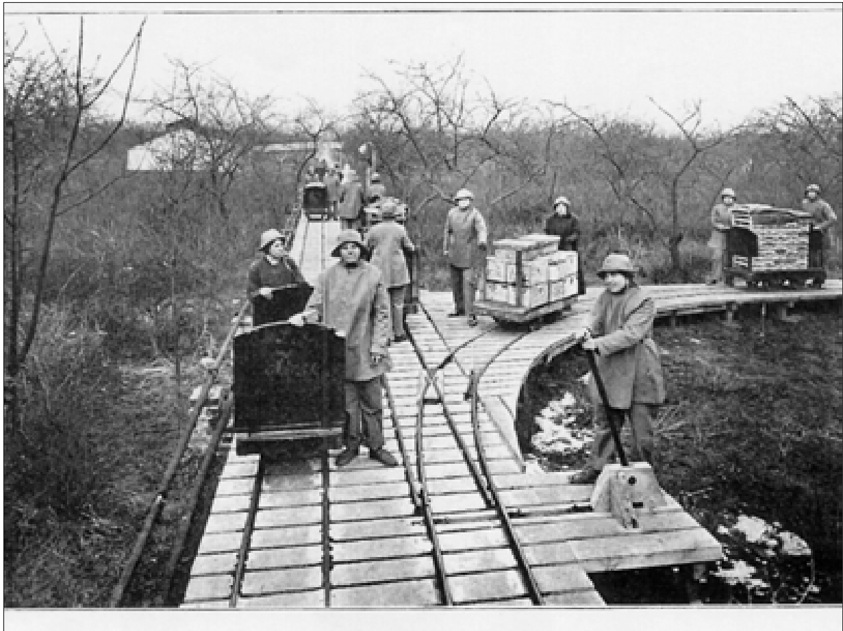
Plate 3: View of walkway and immediate area
