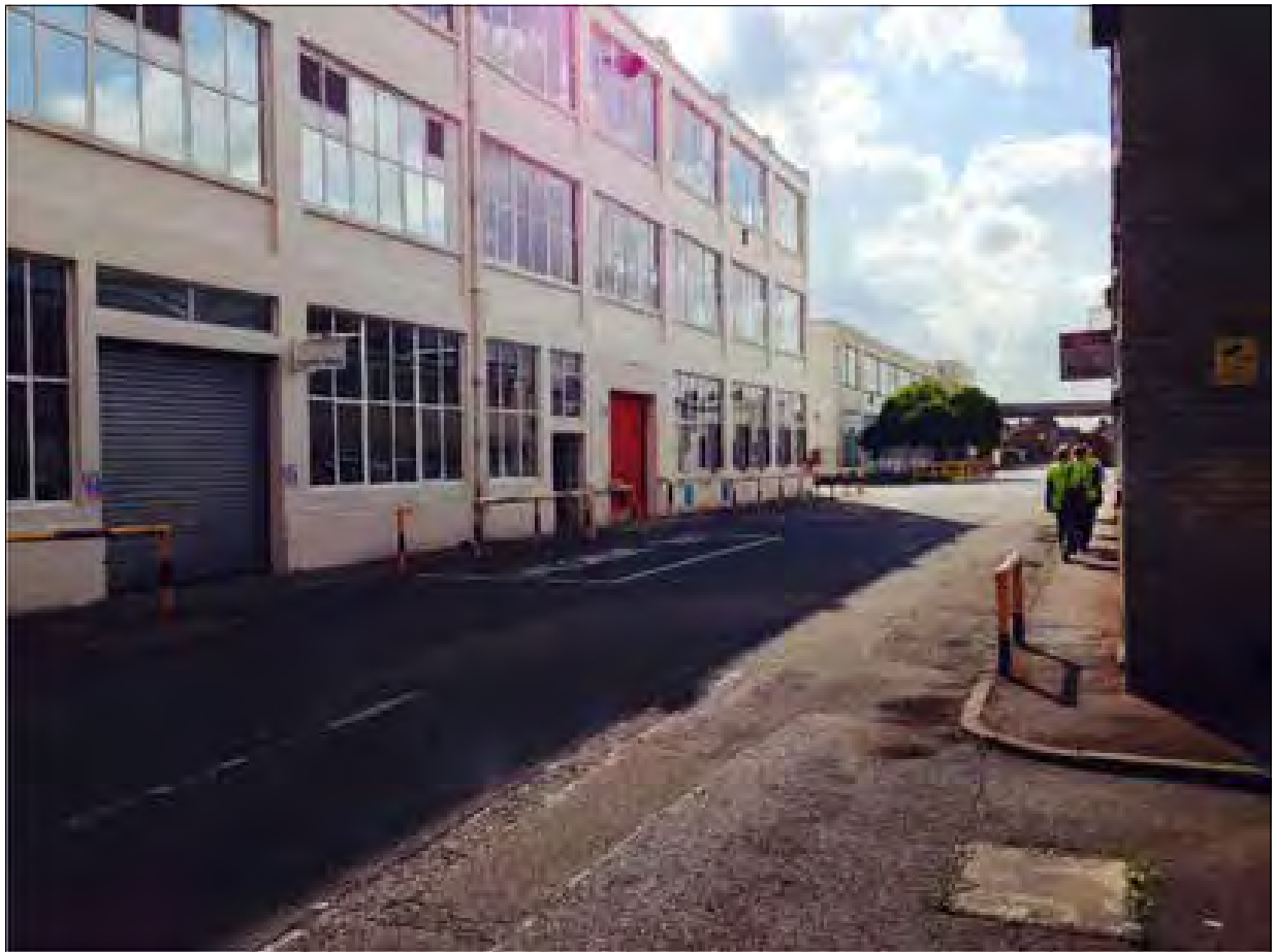
Plate 7: General view of the factory buildings
