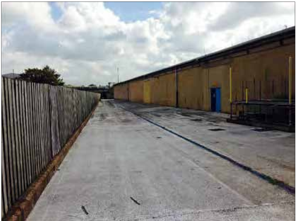
Plate 8: General view of access roads/loading bays
