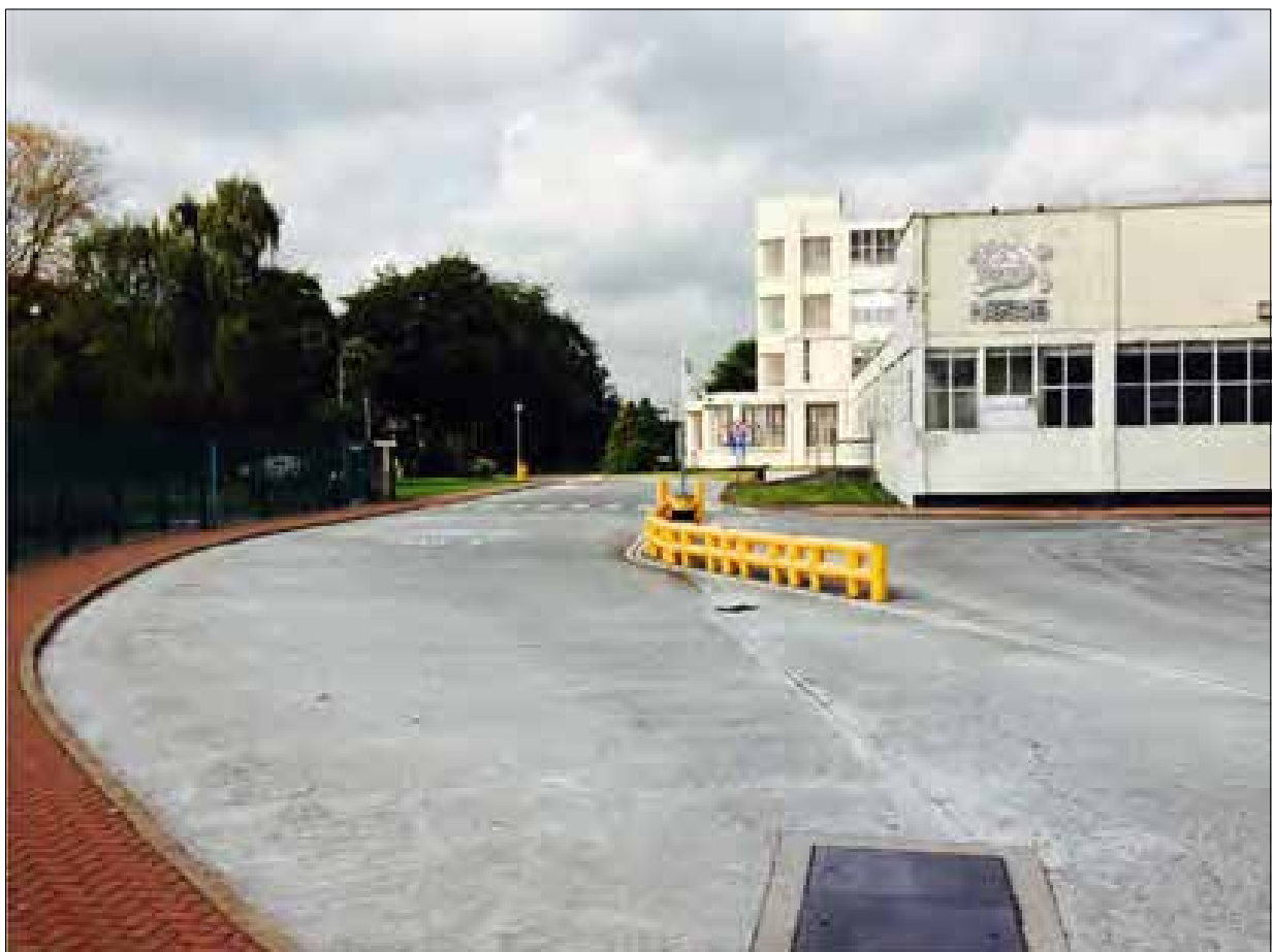
Plate 6: General view of the factory buildings
