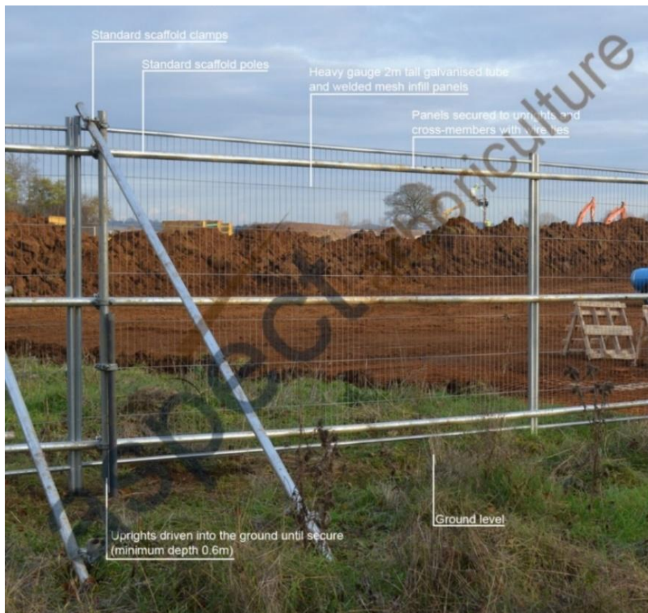
Plate.1 Default Protective Barrier Specification
