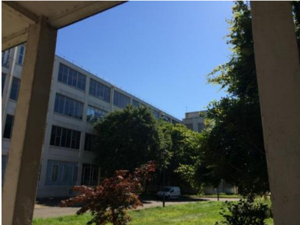
Figure 3.16: The relationship of the locally listed factory building with its later south entrance, the former canteen and the landscaping has some resonance with the interwar intentions for a 'factory in a garden'
