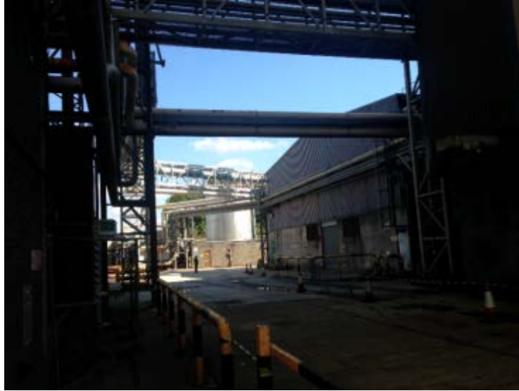
Figure 3.19: View of ad hoc modern additions to the factory which fail to positively contribute to the special interest of the conservation area
