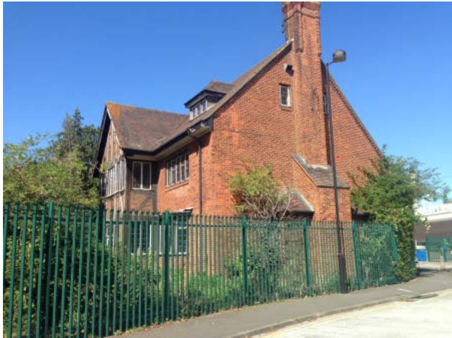
Figure 3.31: View of the east and south façade of the former lodge
