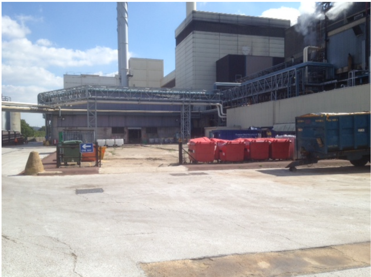
Photograph B8 Former Boiler House Footprint now used as Waste Storage Compound
