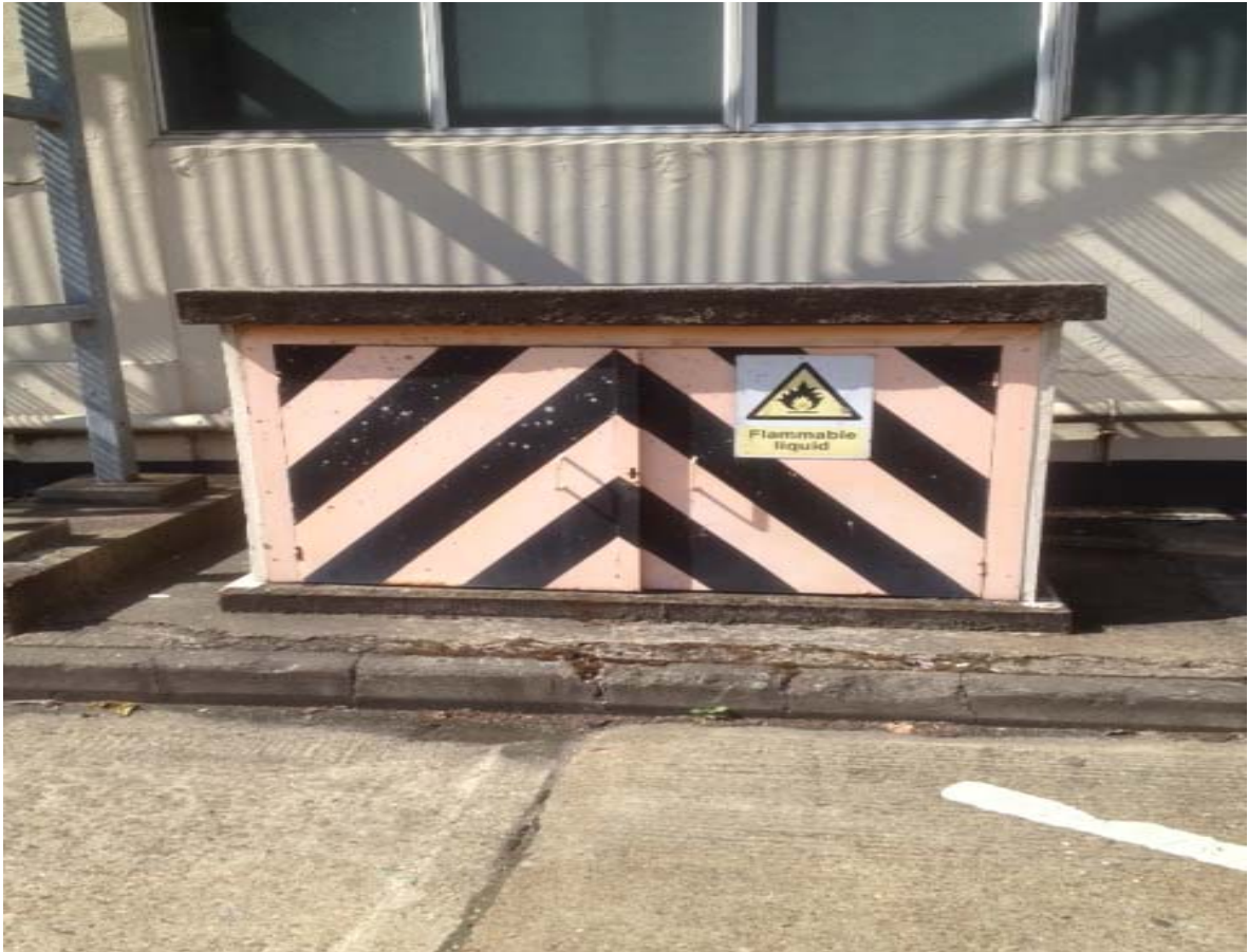
Photograph B3 Example Hazardous Chemical Store
