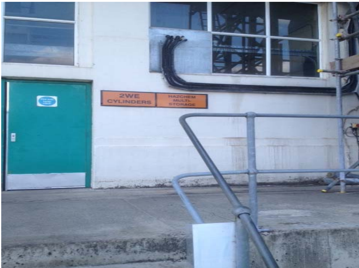
Photograph B4 Entrance to Former Hazardous Chemical Store Close to Boiler House
