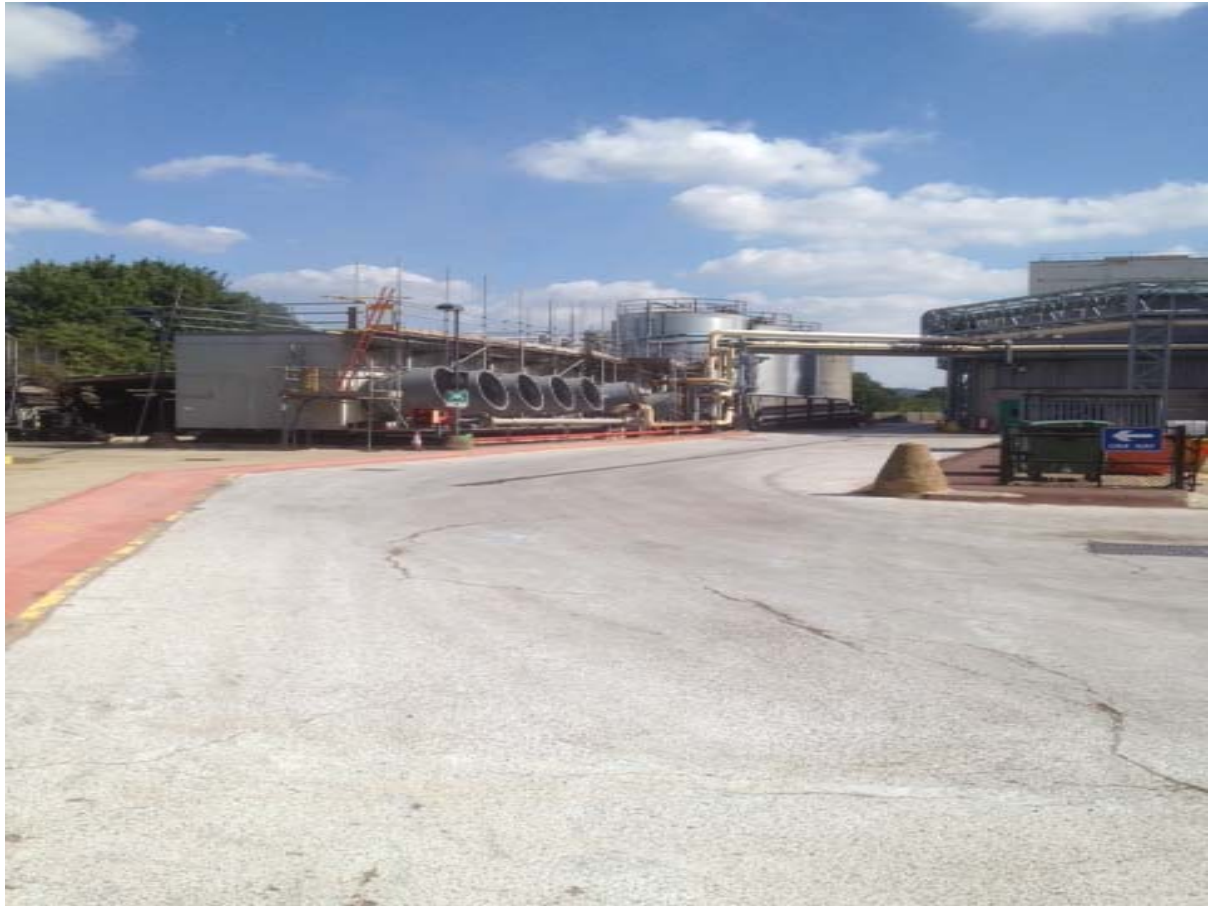
Photograph B9 Distant View of Boiler House, Former HFO Tanks and Cooling Towers
