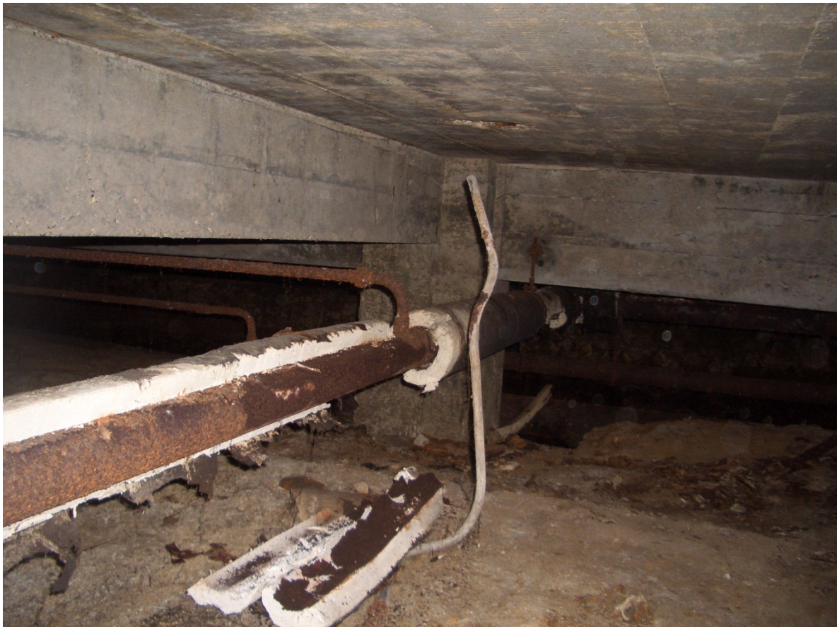
Photograph C4 Undercroft Pipe Lagging
