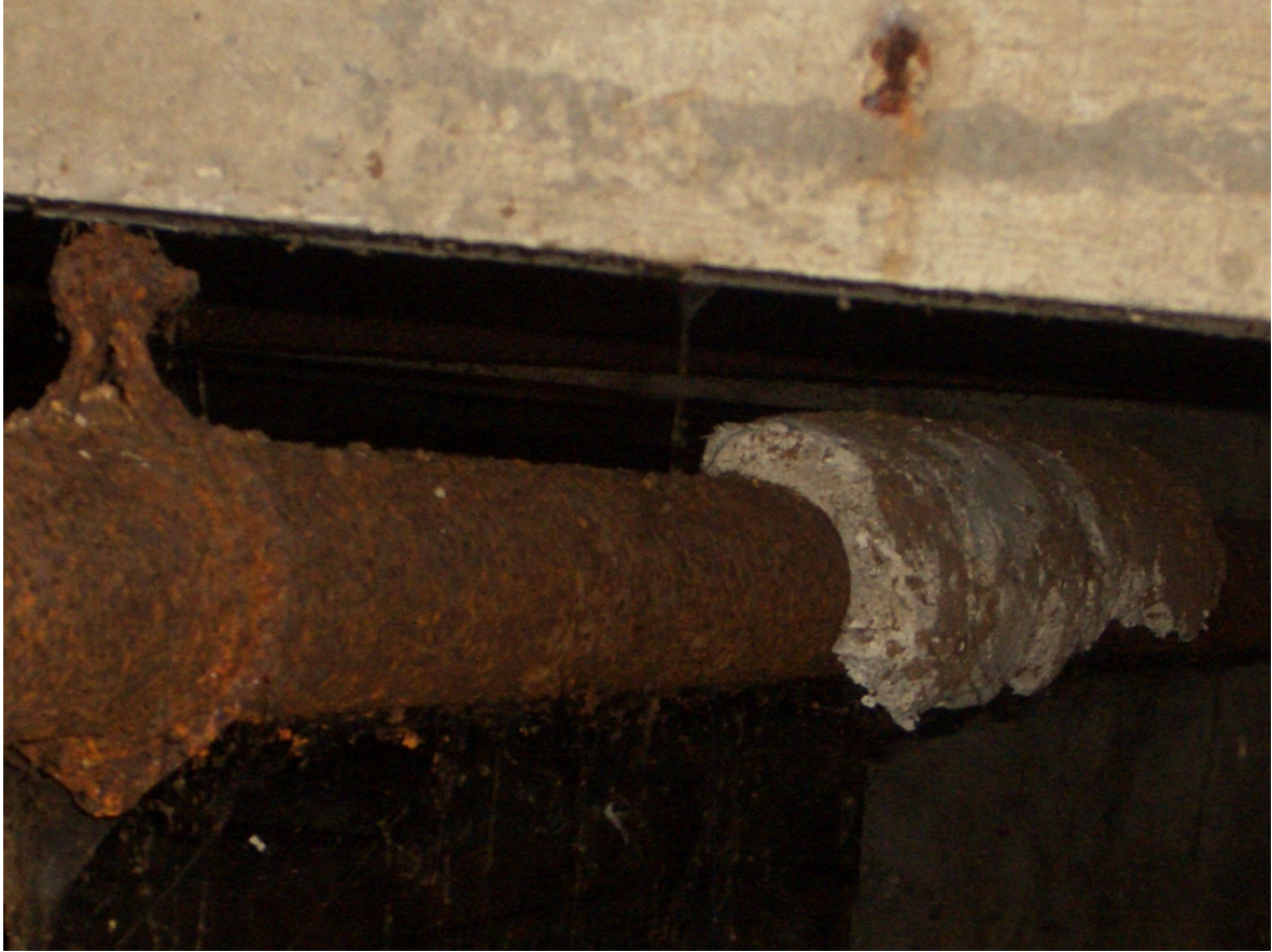
Photograph C3 Undercroft Pipe Lagging
