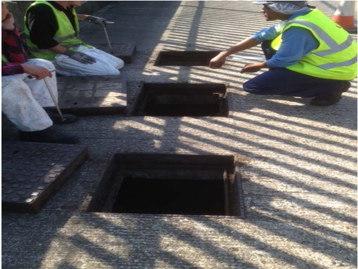
Photograph B5 Oil-Water Interceptor at Eastern Extremity of Site
