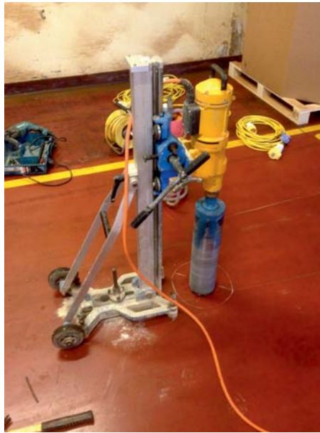
2) Service clearance and coring setup
