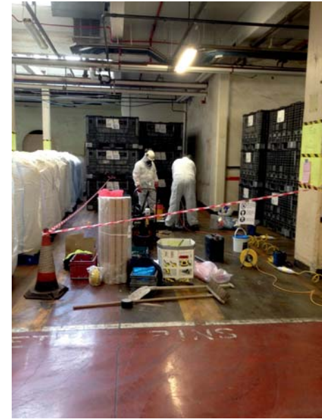
3) Window sampling (drilling) of location
