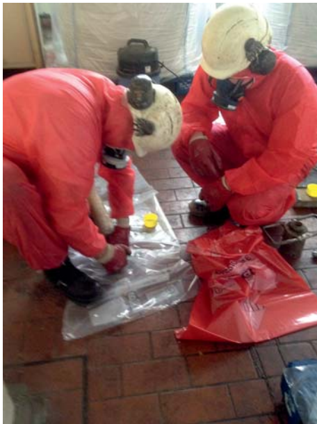
4) Decontaminating of drilling equipment
