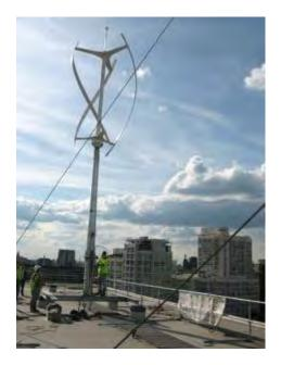
In urban areas non-laminar wind flow occurs as a result of turbulence due primarily to adjacent buildings. There is growing evidence of urban wind turbines failing to perform in line with manufacturer's estimated outputs and as a result wind turbines are likely to produce only modest power outputs with corresponding low carbon dioxide emission reduction within urban sites.
