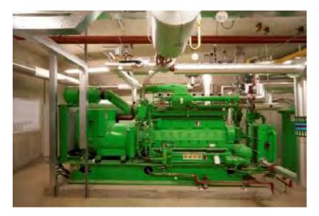
Combined Cooling, Heat and Power (CCHP) that is often referred to as trigeneration uses the same principles as detailed above for a CHP system however the heat produced is also used to generate cooling via an absorption chiller. The CCHP plant can make use of heat generated by the CHP plant in buildings with a cooling demand.
