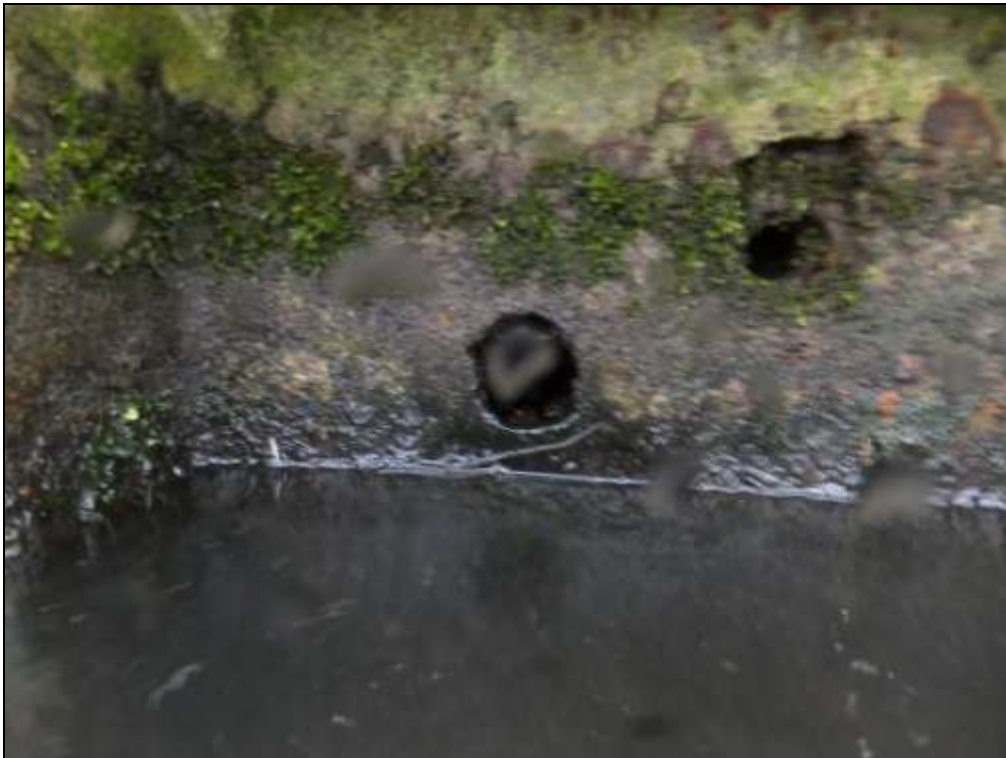
Photograph 28: Ch 180m – 2# holes.
