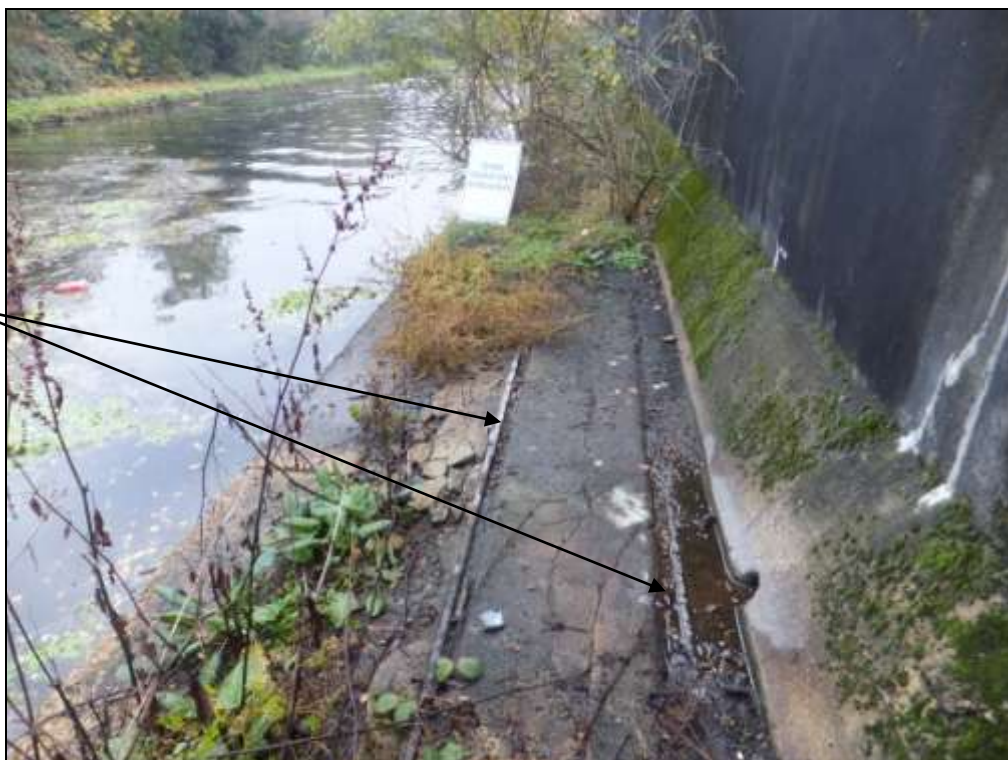
Photograph 38: Ch 241m – Cracking to corner section of capping beam.
