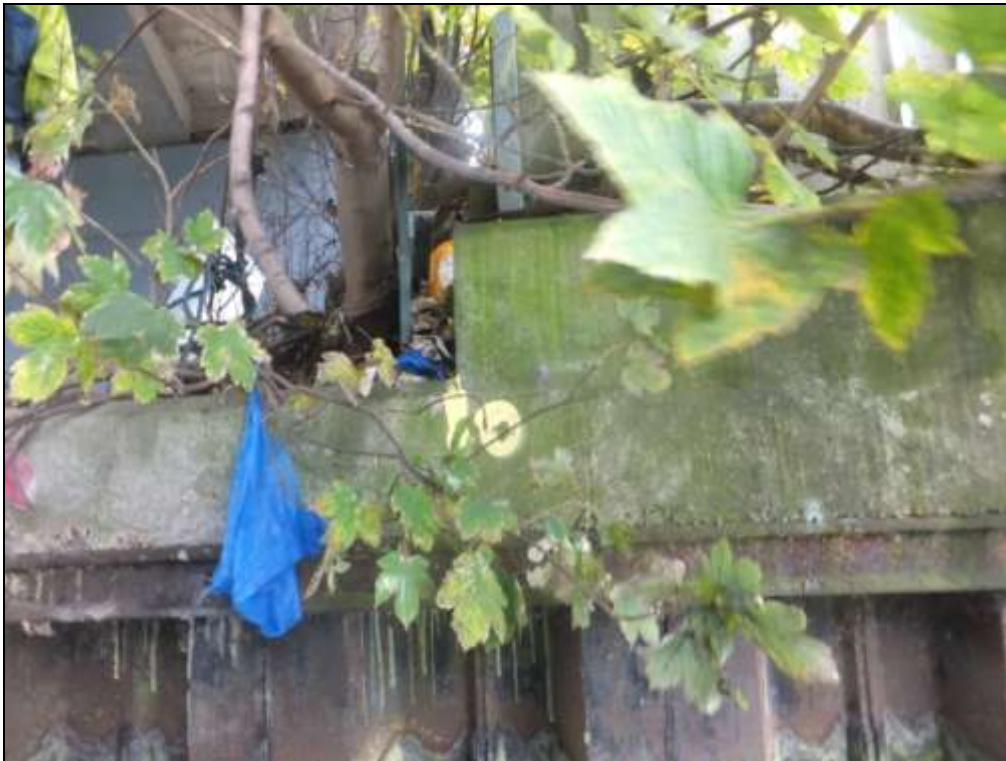
Photograph 1: Ch 0m – Location picture of chainage 0m.
