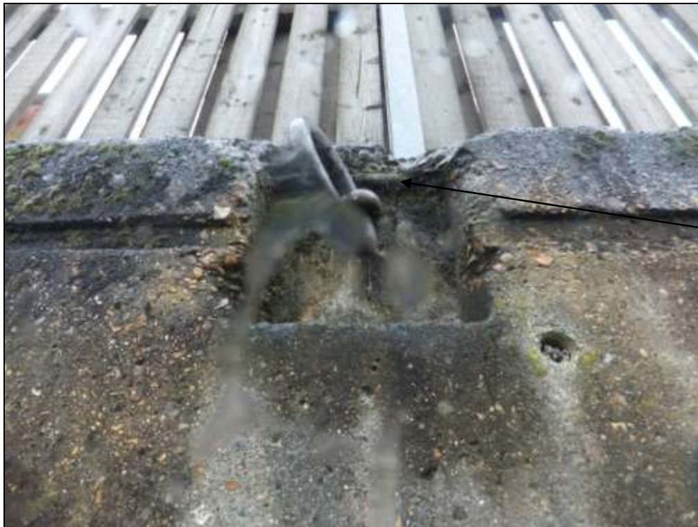
Photograph 11: Ch 65m – Damage to mooring ring recess with re-bar exposed.
