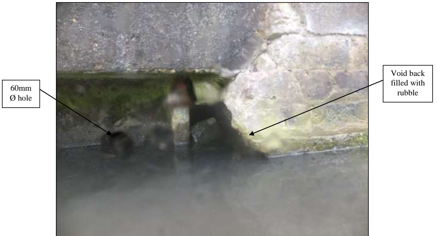
Photograph 32: Change in construction to Larssen No. 2 sheet piles.
