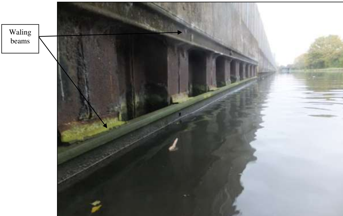
Photograph 2: Ch 0m – 9m – Initial 9m of the unknown sheet pile.
