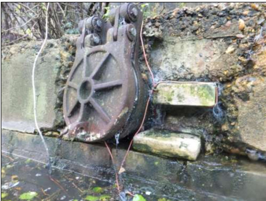
Photograph 42: Ch 287m – Outfall pipe with flap valve.
