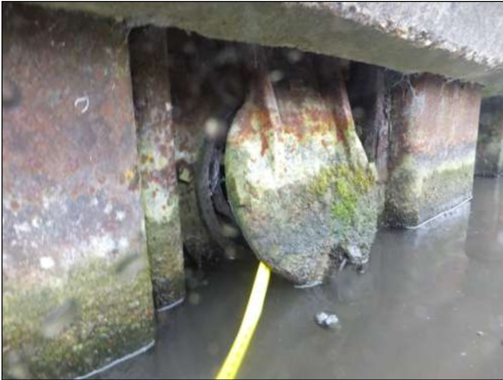
Photograph 15: Ch 39.5m – Outfall pipe with operational flap valve.
