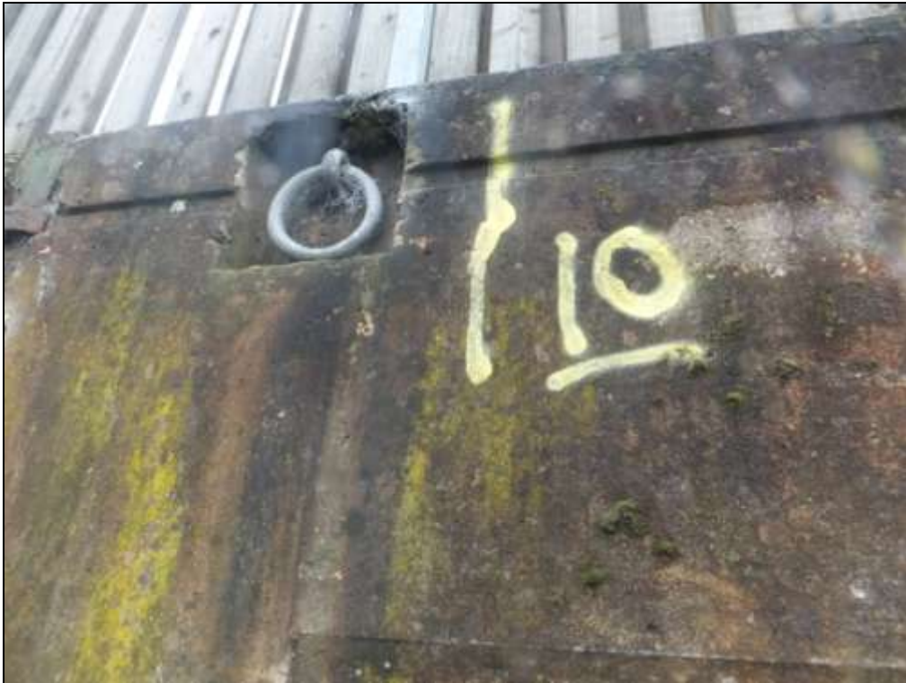
Photograph 9: Ch 10m – Mooring ring recessed into the capping beam.
